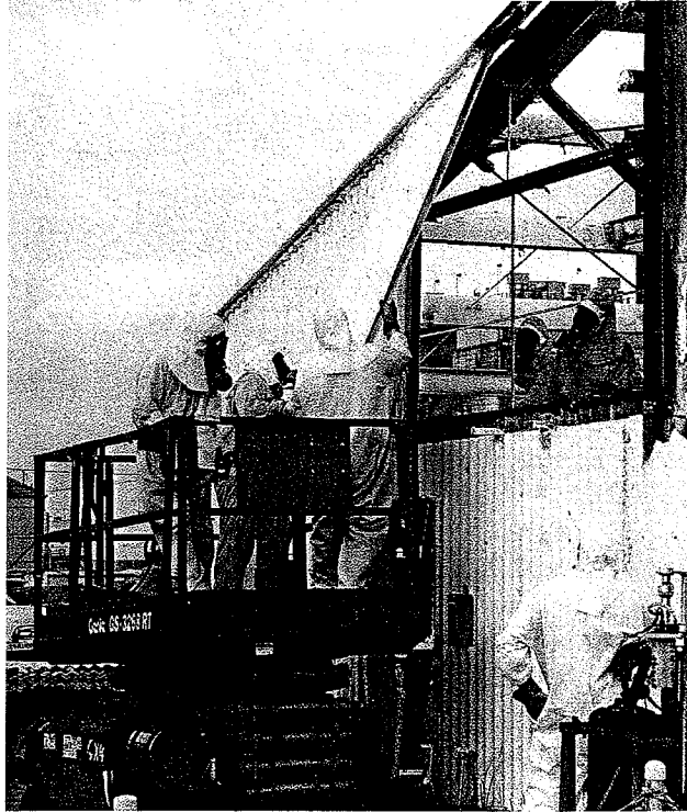
Figure 5. Photograph of Transite Siding Removal at C-405
