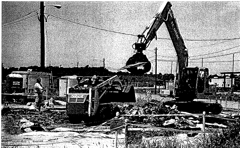
Figure 8. Photograph of Site Cleanup at C-405
