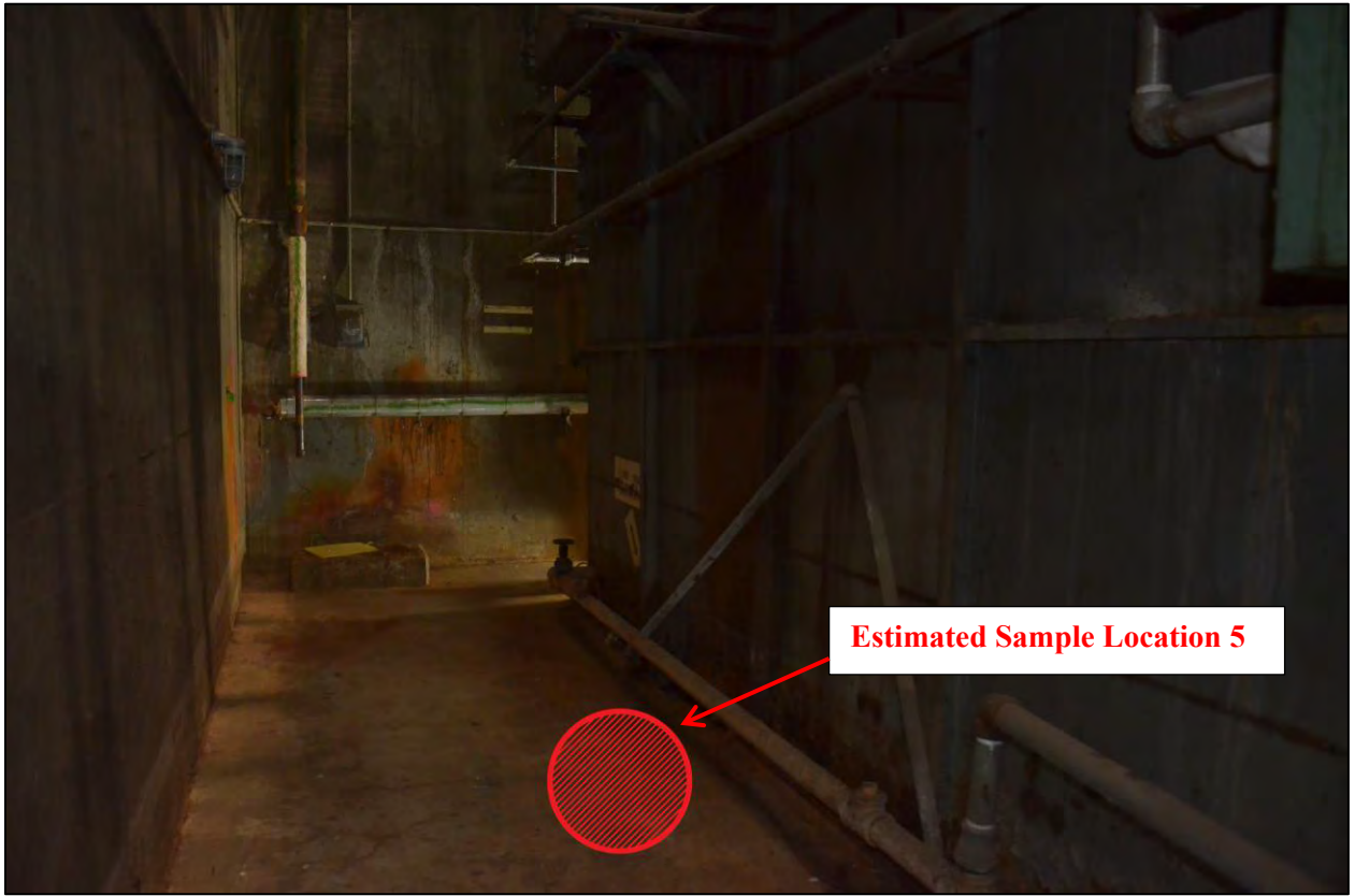
Figure D.5. Sampling Location 5, Basement Level Near Degreaser Tanks
