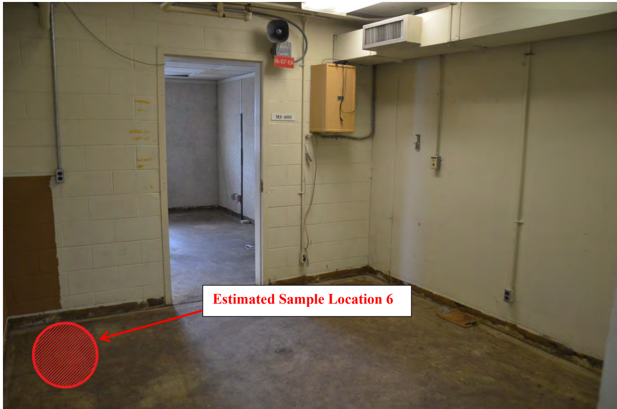
Figure D.6. Sample Location 6, Southeast Office
