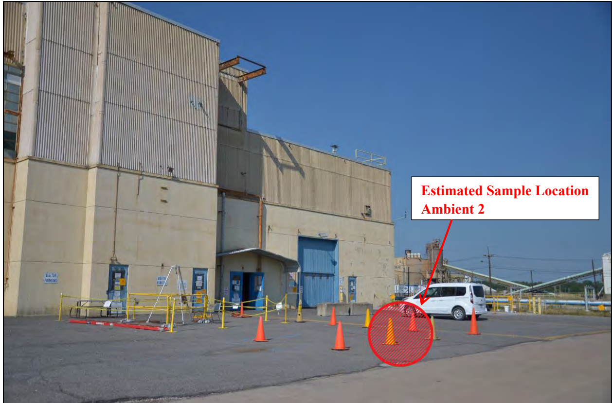
Figure D.10. Sample Location Ambient 2, North Location, 50 ft North of Building
