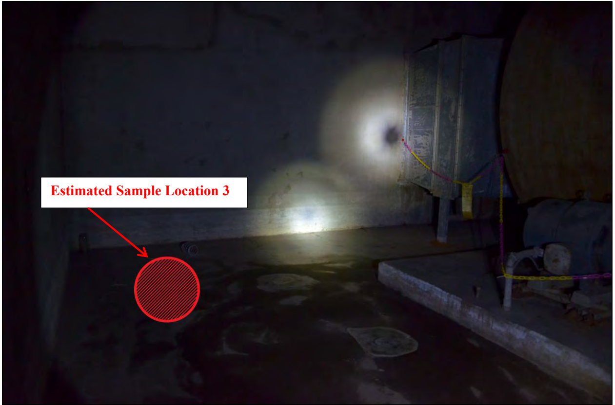
Figure D.3. Sample Location 3, Basement Furnace Room on North End
