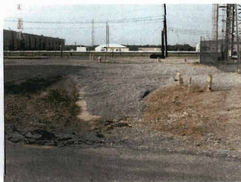
Fig. 1.5. View of Sector 4 (Southeast) including SWMU 11—TCE Leak Site
