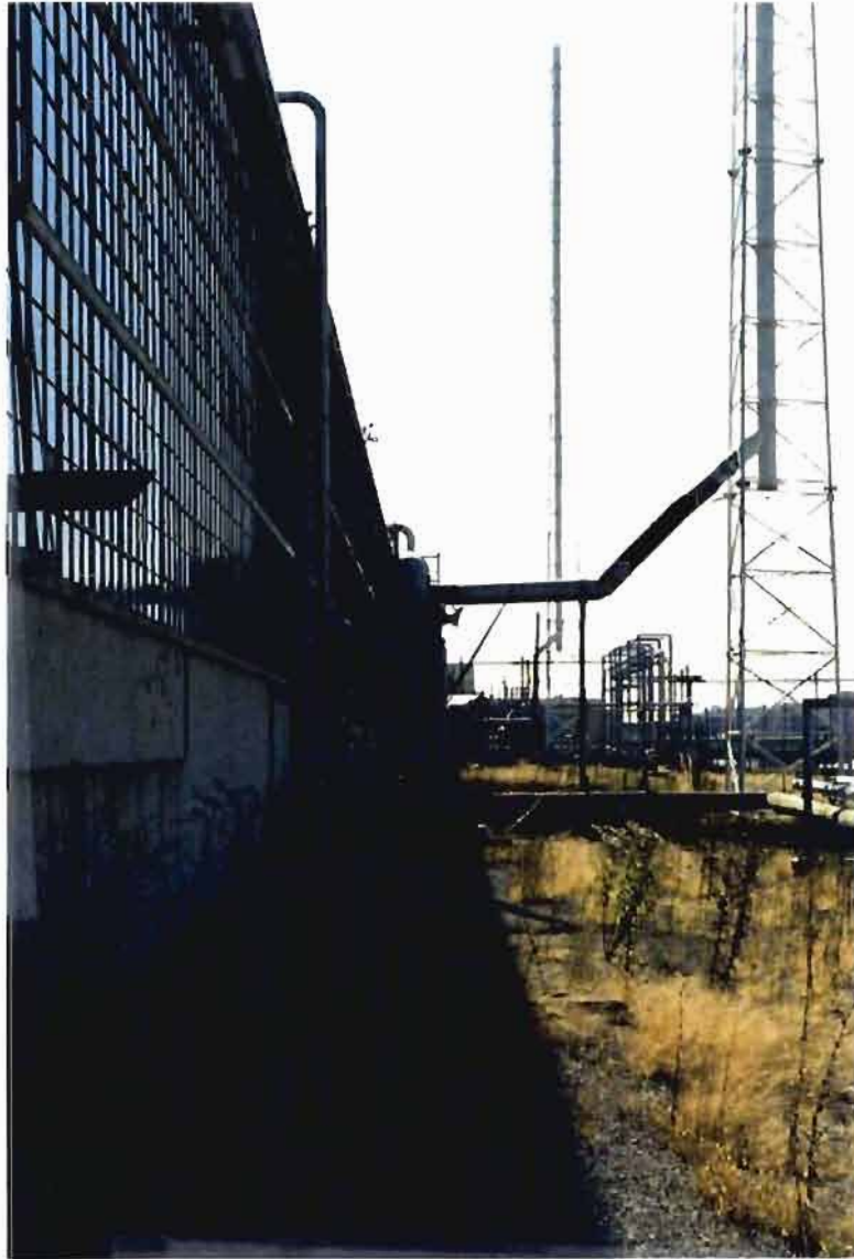
5. Nitric Acid Scrubber
