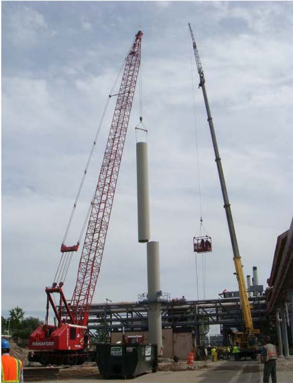
Figure A.10. Stack Demolition (Crane Assisted and OSHA Basket)
