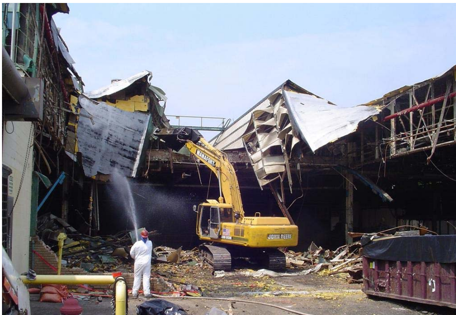
Figure A.3. Building Structure and Roof Demolition (Shear and Fugitive Dust Control)
