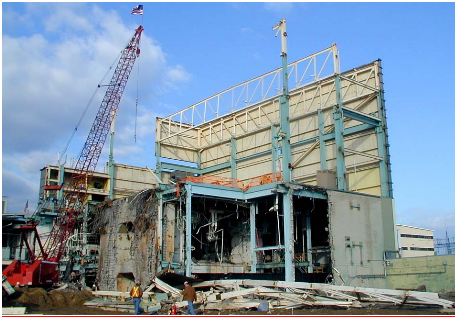
Figure A.7. High Bay Roof Truss Removal (Crane Assisted Disassembly)
