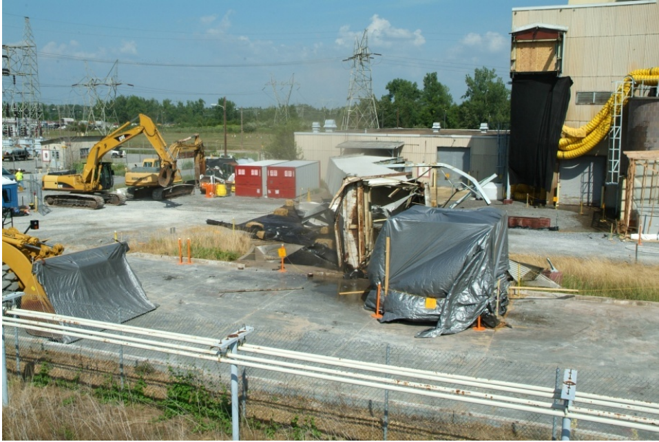
Figure A.13 C-340 Complex Conveyer Structure on the Ground
