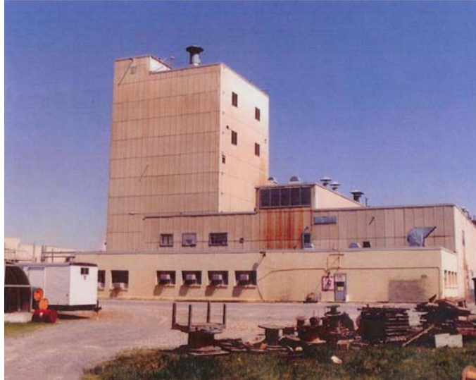
Figure 2. Exterior of the C-340 Complex
