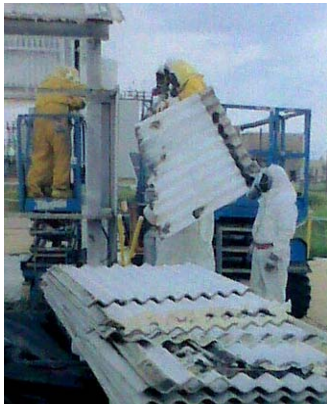
Figure A.5. Transite Siding Removal and Packaging
