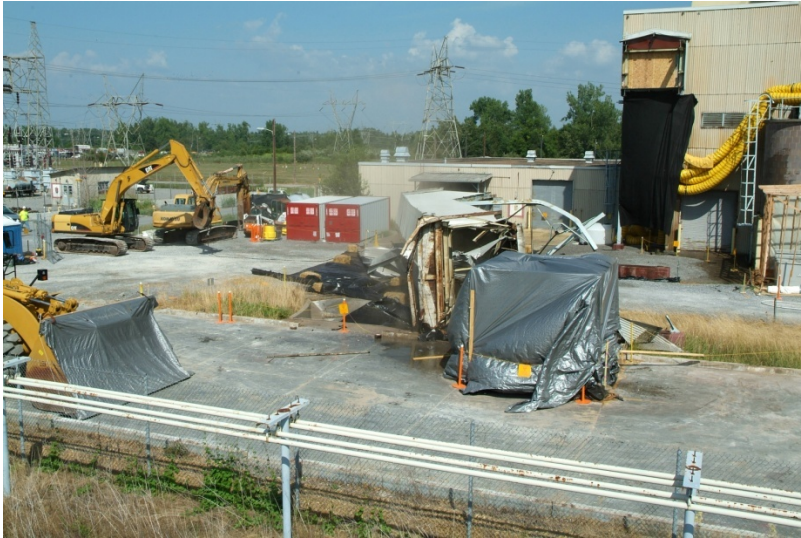
Figure A.13 C-340 Complex Conveyor Structure on the Ground
