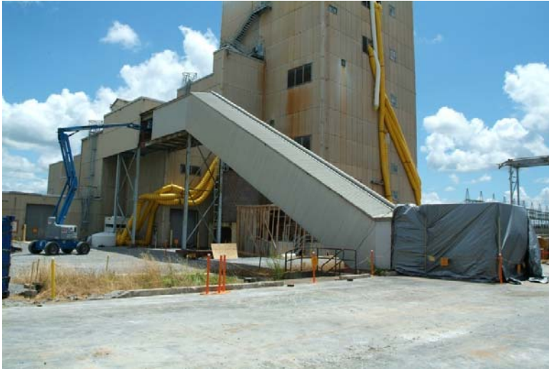
Figure A.11. C-340 Complex Conveyor Prior to Demolition (Personnel are accessing the conveyor structure from the man-lift to disconnect the conveyor from the building.)
