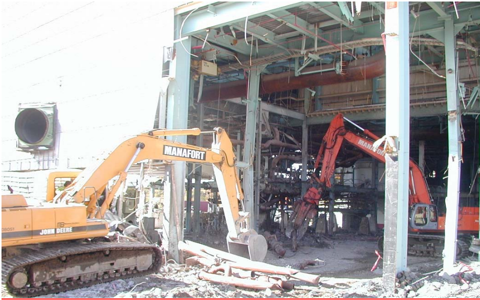
Figure A.4. Interior Building Mezzanine and Equipment Removal Prior to Demolishing the Structure
