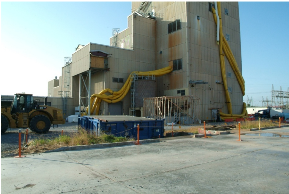
Figure A.14. C-340 Complex Area Following Cleanup and Packaging of Debris from the Conveyer Demolition
