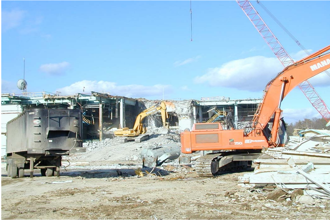
Figure A.8. High Bay Roof Trusses and Columns Removed
