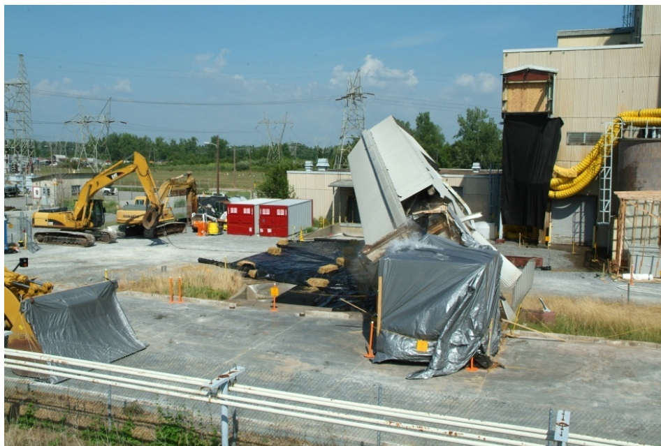
Figure A.12. C-340 Complex Conveyor Being Pulled Over by Excavator (The conveyor was cut away from the building prior to being pulled over. The plastic on the ground collects dust from the structure when it contacts the ground.)
