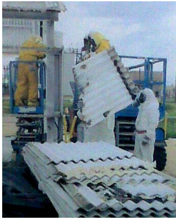
Figure A.5. Transite Siding Removal and Packaging
