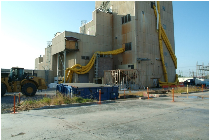
Figure A.14. C-340 Complex Area Following Cleanup and Packaging of Debris from the Conveyor Demolition
