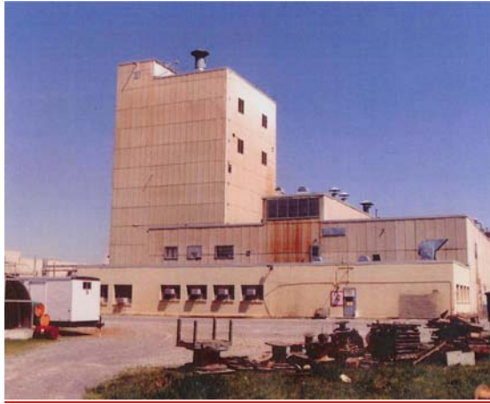
Figure A.2. Exterior view of the C-340 Metals Reduction Plant Complex
