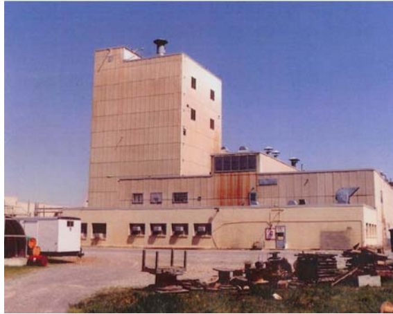
Figure 2. Exterior of the C-340 Complex
