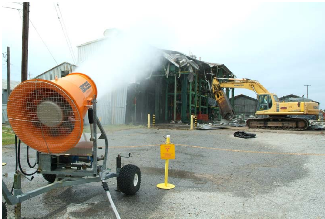
Figure A.15. Demolition of the C-746-A East End Smelter Showing Use of a Dust Boss to Reduce Dust Generation
