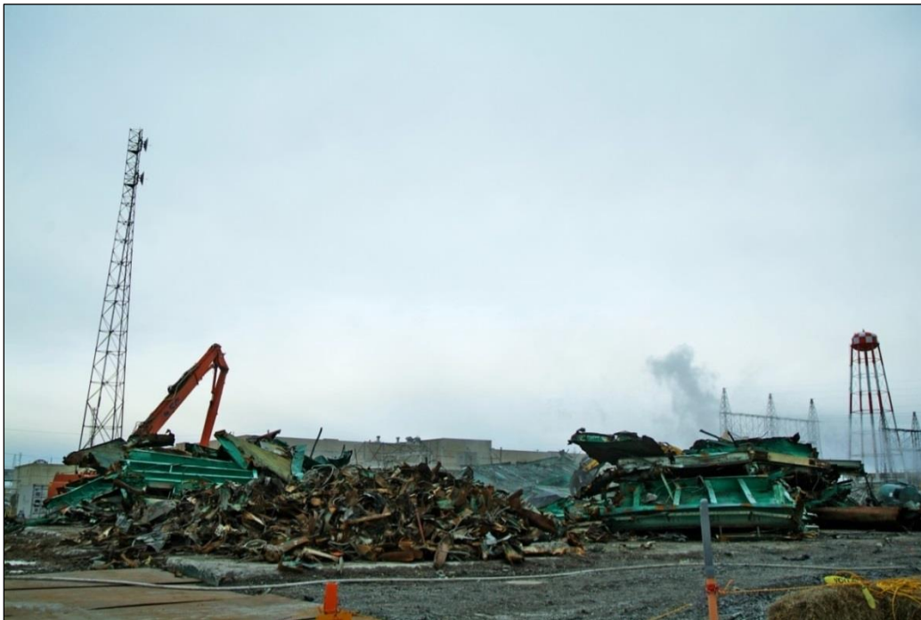
Figure A.14. Debris Being Processed Following Demolition (Debris segregated from different parts of building by sequencing demolition; separate debris piles maintained for landfill disposal and off-site shipment.)
