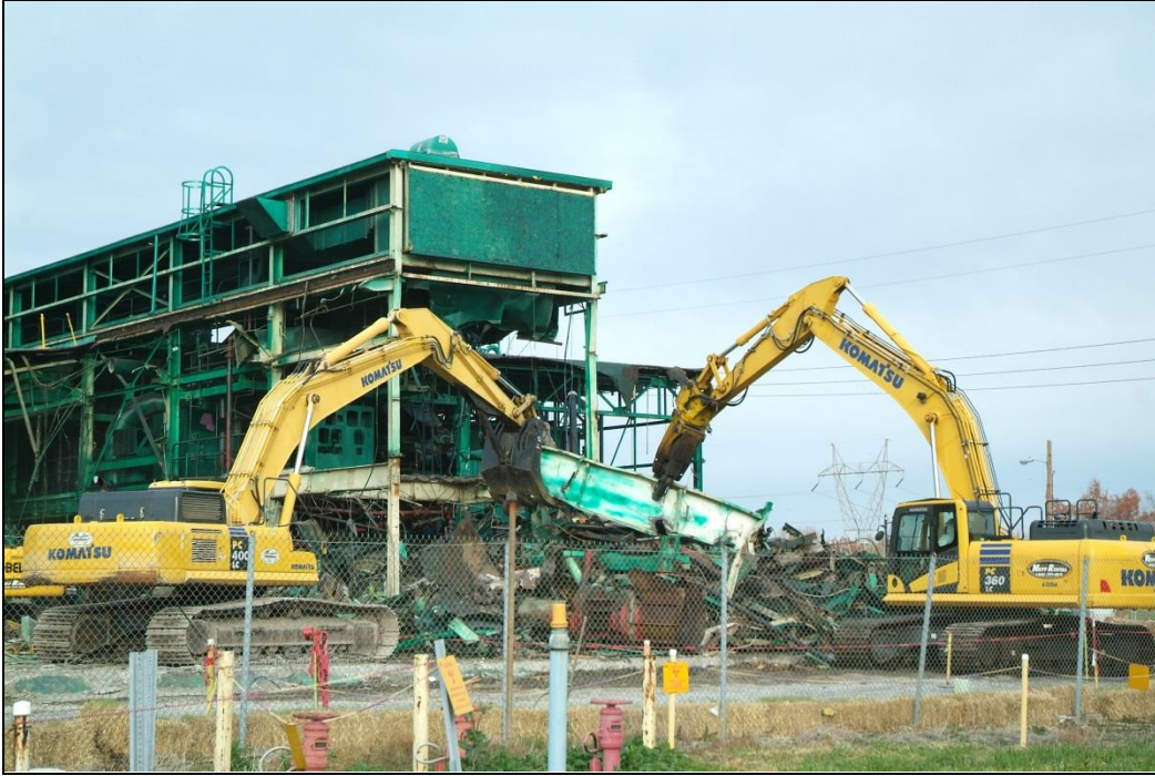
Figure A.9. Two Excavators Downsize a Beam from the C-340-B Metals Plant Building (Debris from this building loaded in gondolas for off-site shipment.)
