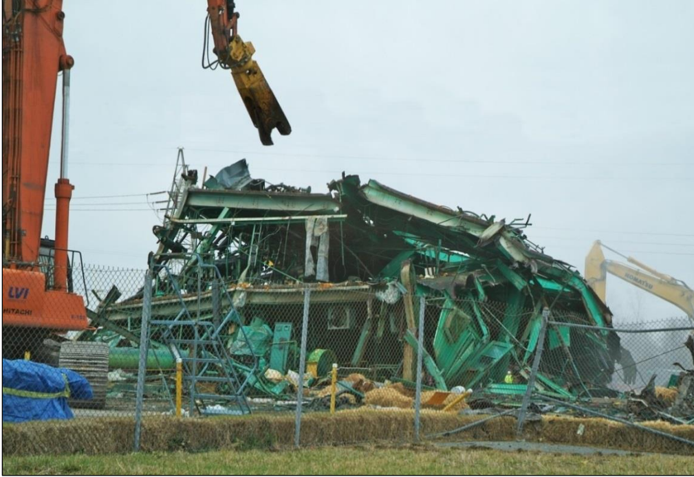
Figure A.13. The Support Beams for the Metals Plant Are Cut To Bring the Building to Slab
