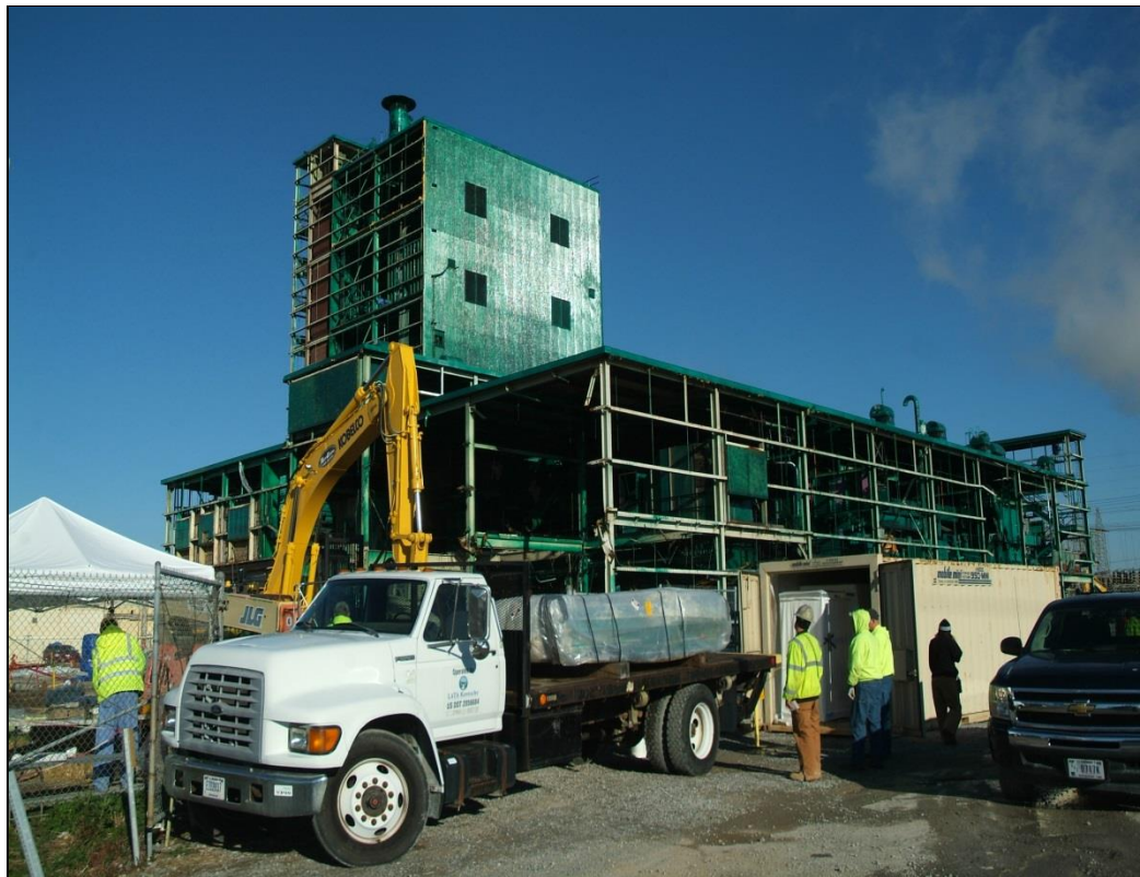
Figure A.6. Double-wrapped Stacks of Transite Panels Are Loaded on Truck for Transport
