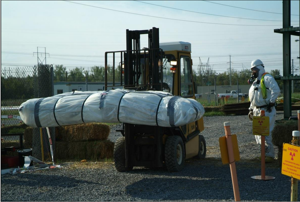
Figure A.5. Double-wrapped Stack of Transite Panels Are Moved to Loading Area
