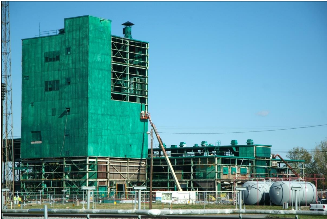
Figure A.2. A Man-lift Is Used to Reach Fixative-sprayed Transite Panels
