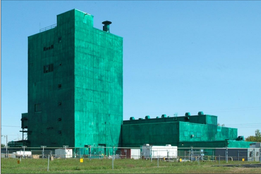
Figure A.1. C-340 Complex Prior to Demolition
