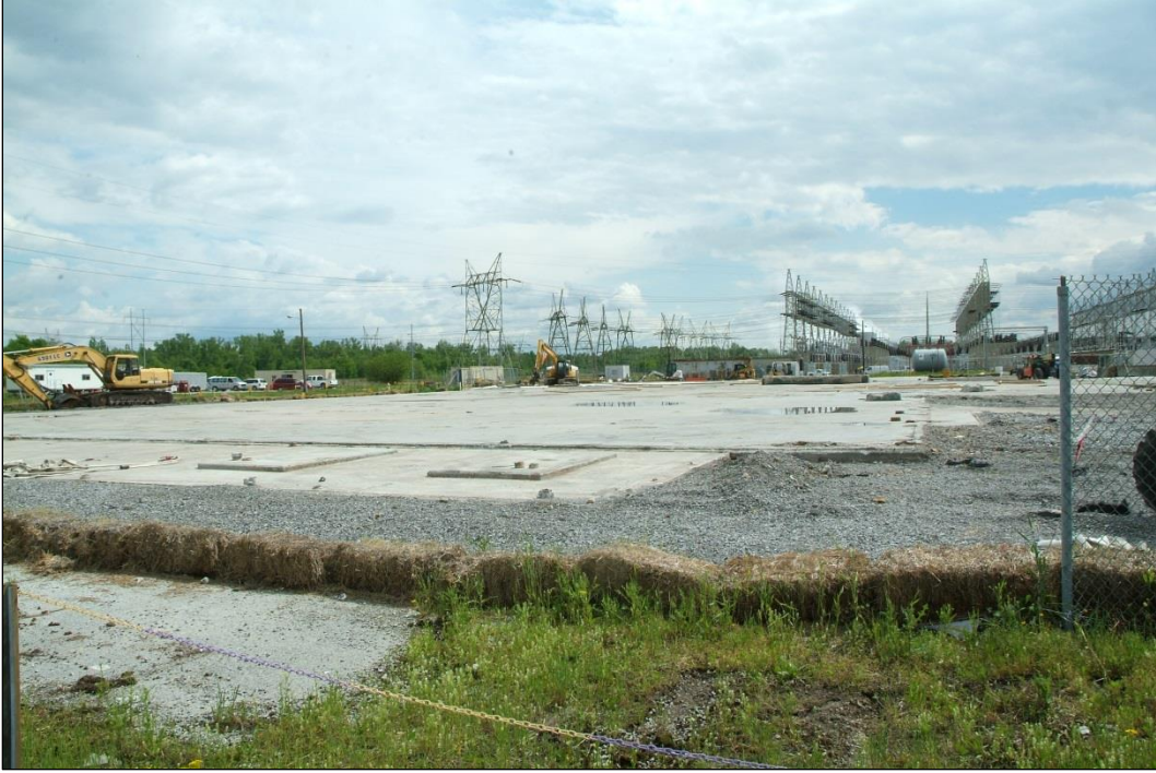
Figure A.15. C-340 Complex after Demolition
