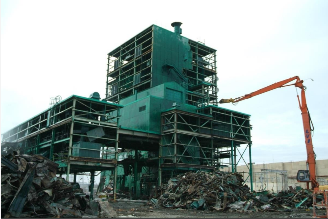
Figure A.11. An Ultra-high-reach Demolition Machine Is Used To Remove Parts of the Building That Can't Be Reached by the Smaller Excavators
