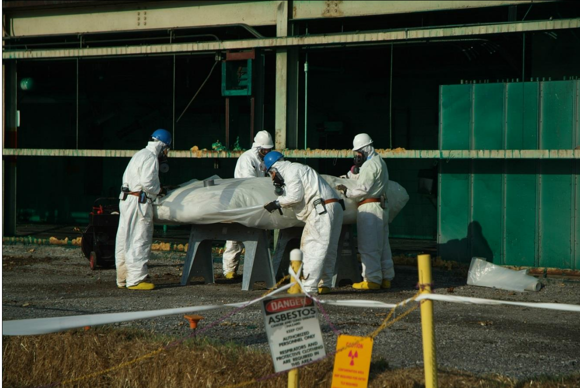
Figure A.4. Workers Wrap Stacked Transite for Disposition
