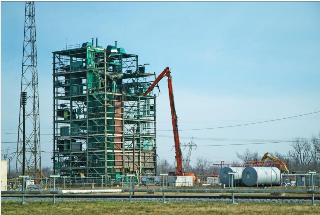
Figure A.12. An Ultra-high-reach Demolition Machine Is Used to Demolish the Metals Plant from the Top Down
