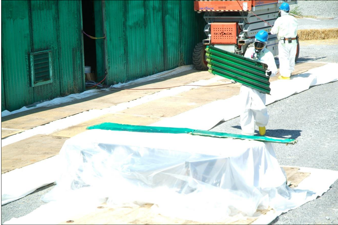
Figure A.3. Workers Stack Removed Transite on Plastic Sheeting
