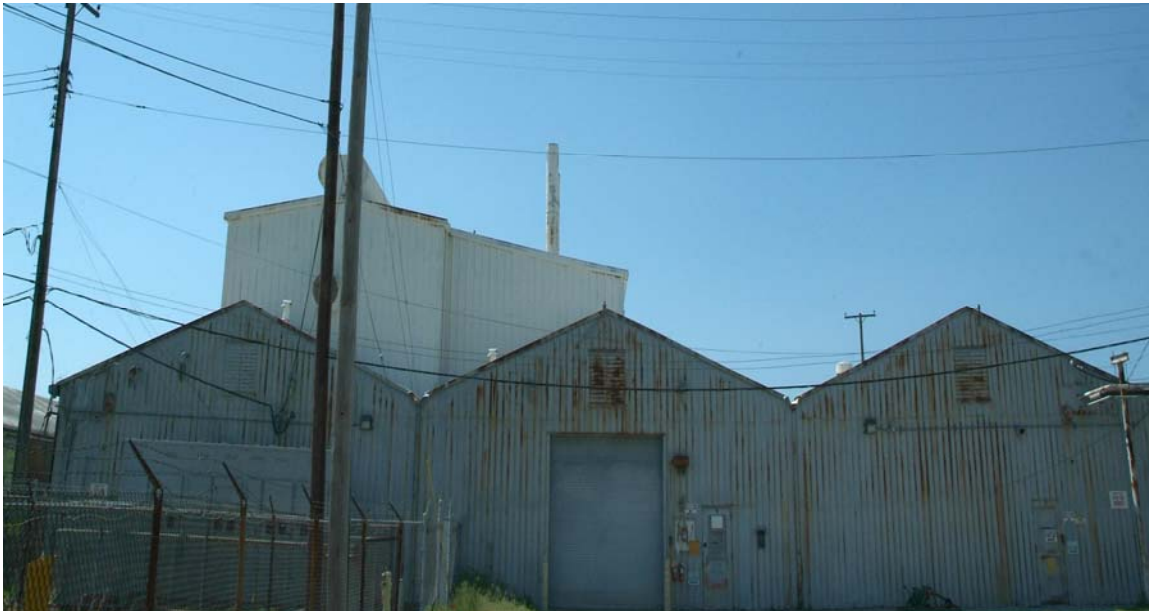
Figure 8. Exterior of the C-746-A East End Smelter
