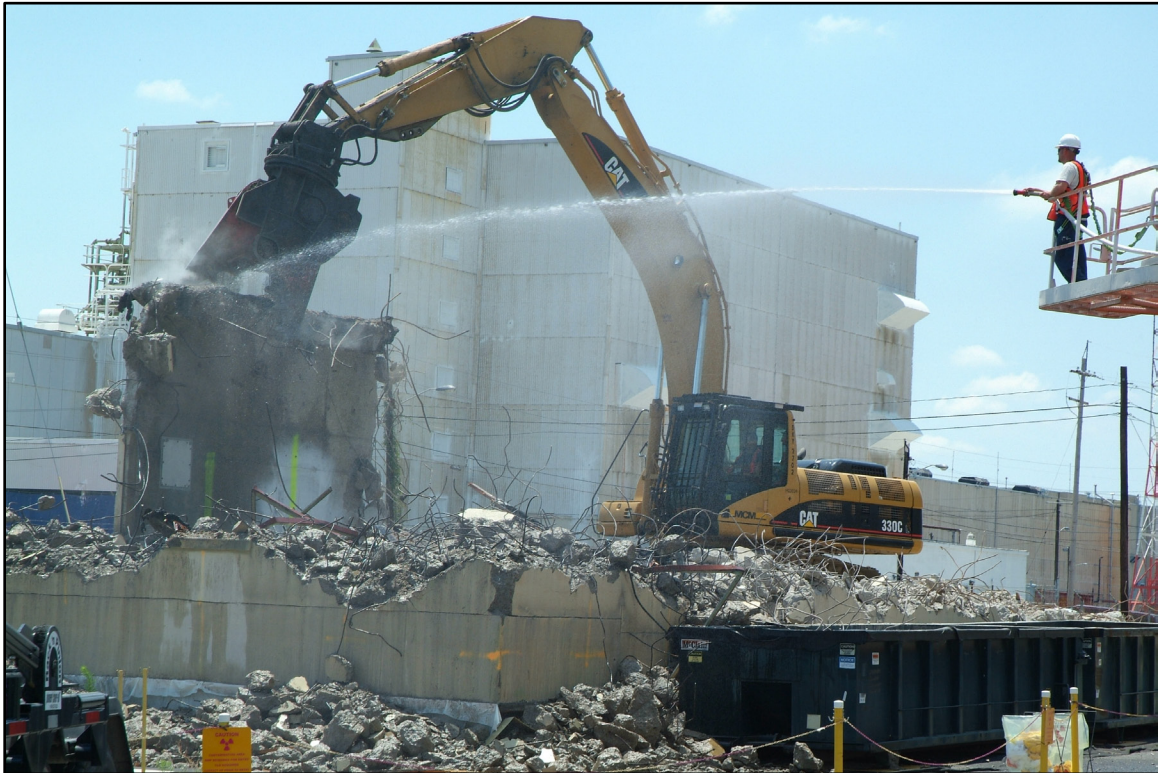
Figure 7. Using a Fire Hose for Dust Suppression during Building Demolition
