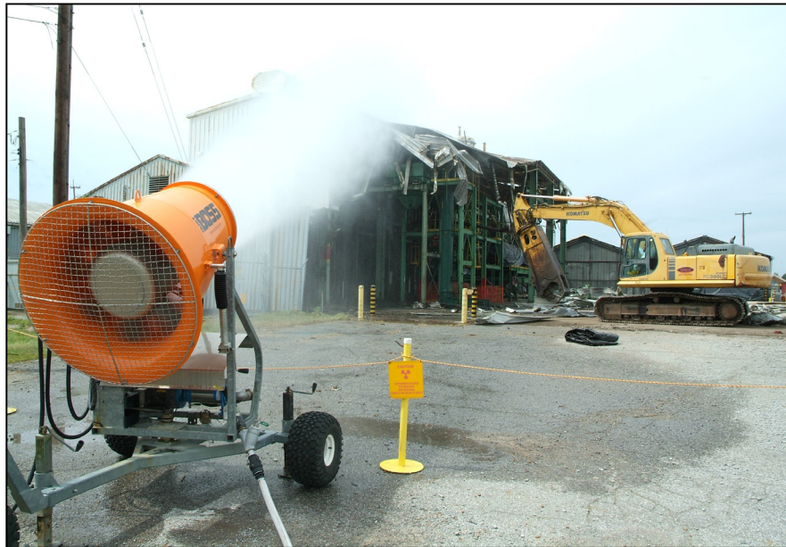
Figure 6. A DustBoss ® Being Used for Dust Suppression
