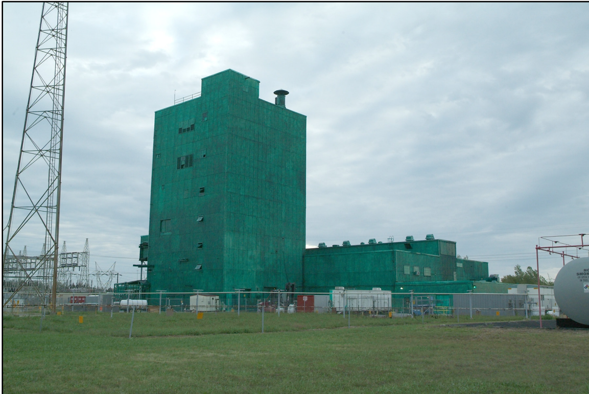
Figure 5. C-340 Complex after Application of ABC® Fiberspray
