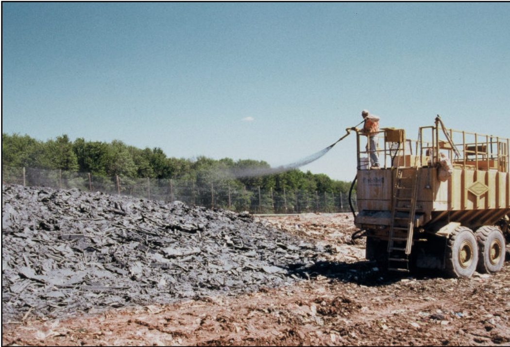
Figure 8. An Example of Applying Alternative Daily Cover at a Landfill
