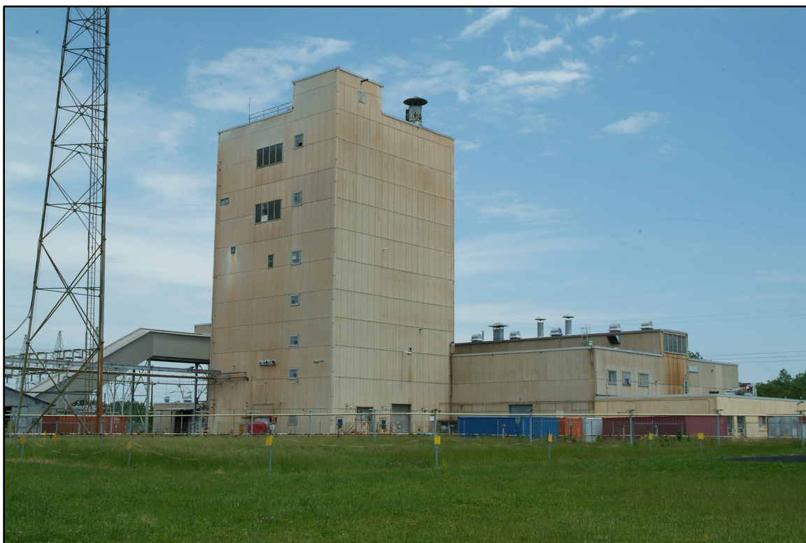
Figure 4. C-340 Complex before Application of ABC ® Fiberspray
