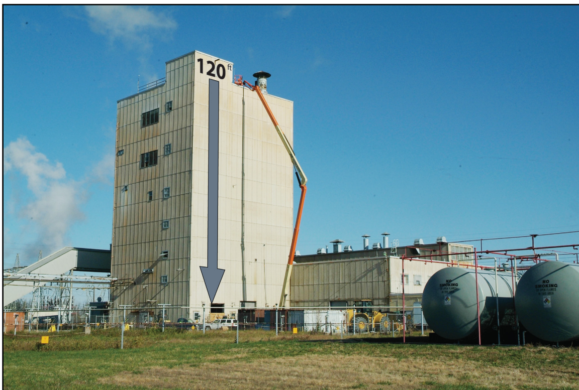
Figure 2. C-340 Building Looking East
