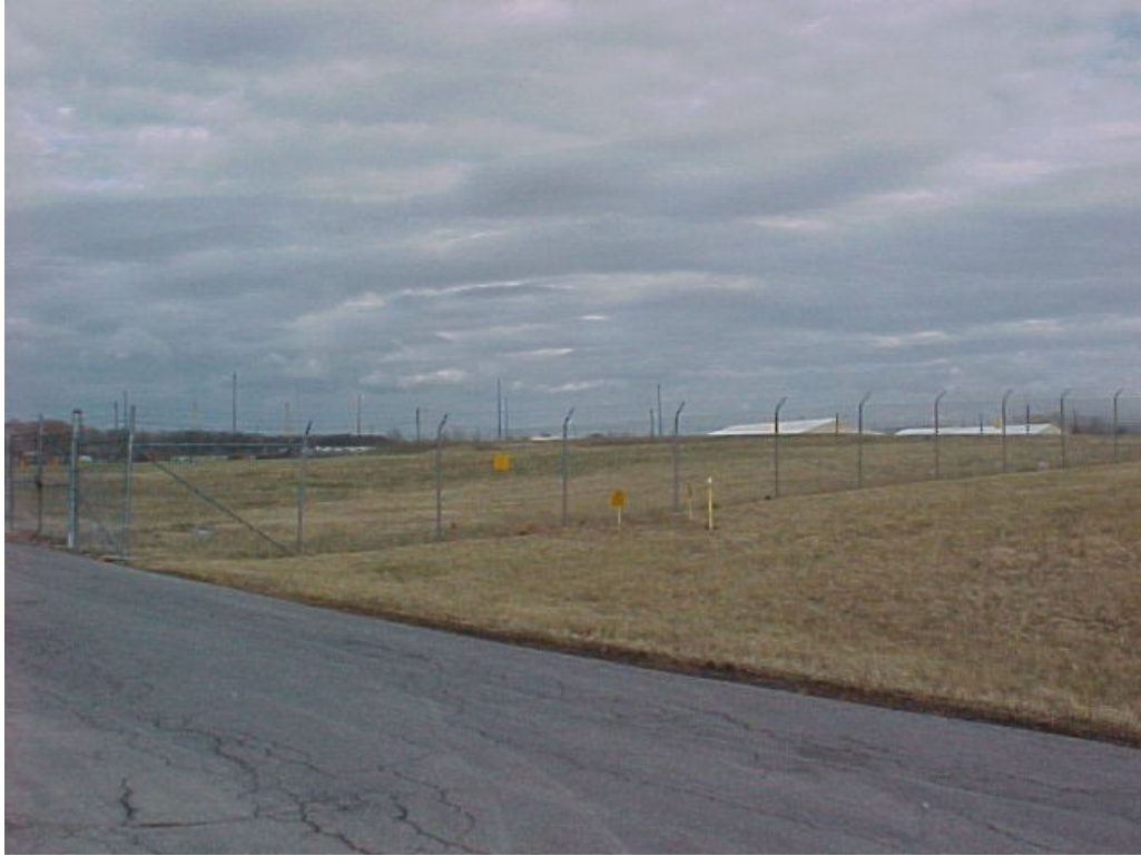
Figure G.4. Surface of SWMU 4 (Area behind Fence)
