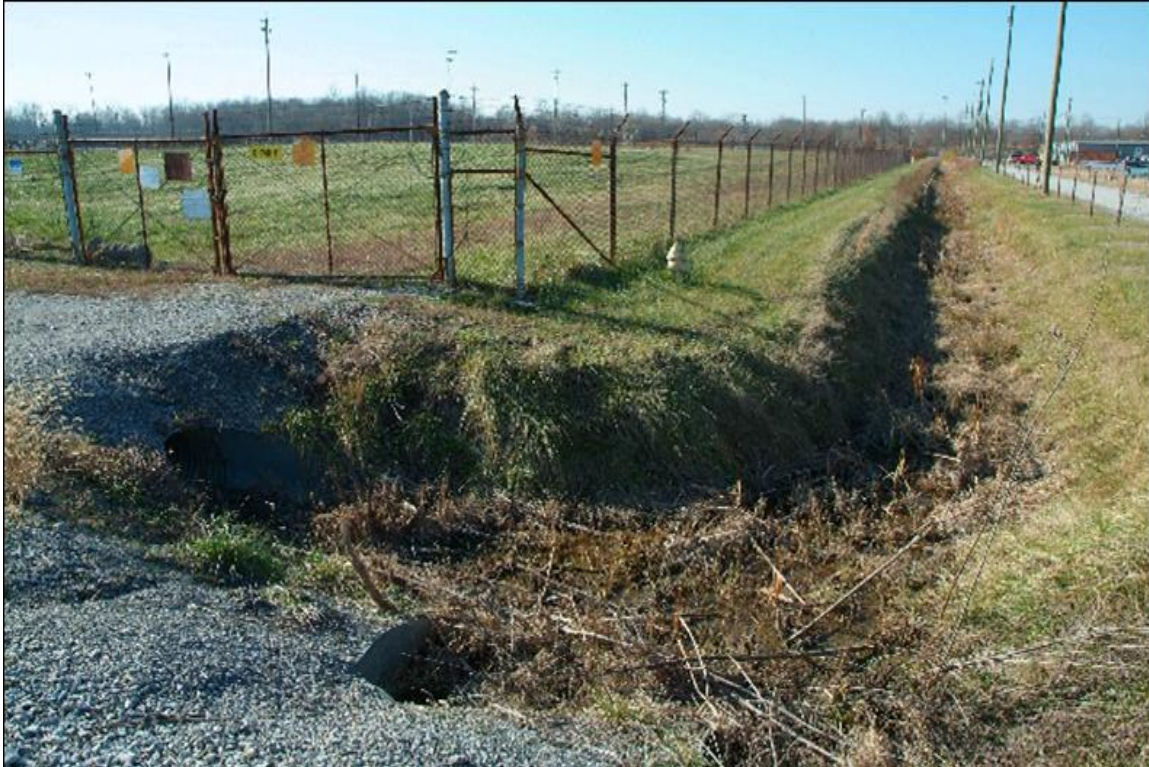
Figure G.5. Surface of SWMU 5 (Area behind Fence)
