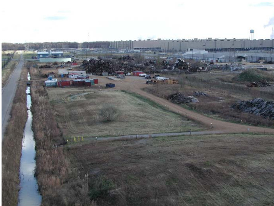
Figure G.7. Surface of SWMU 7 (Field with Tree Surrounded by Road)
