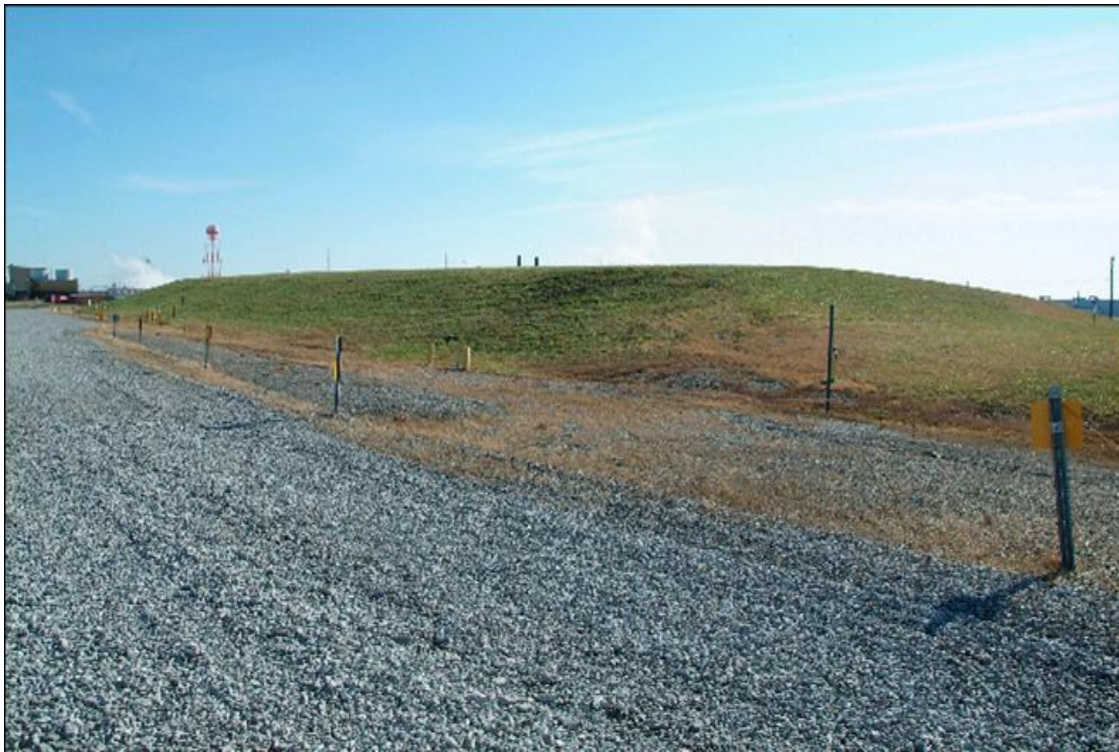
Figure G.3. Surface of SWMU 3
