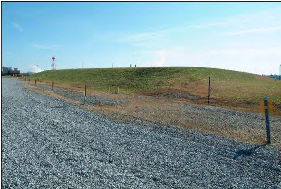
Figure G.3. Surface of SWMU 3
