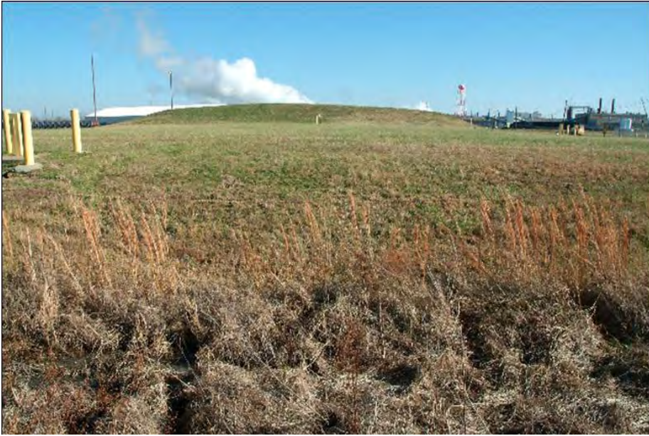
Figure G.2. Surface of SWMU 2
