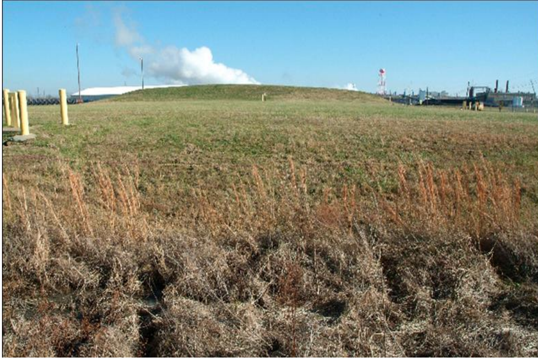
Figure G.2. Surface of SWMU 2
