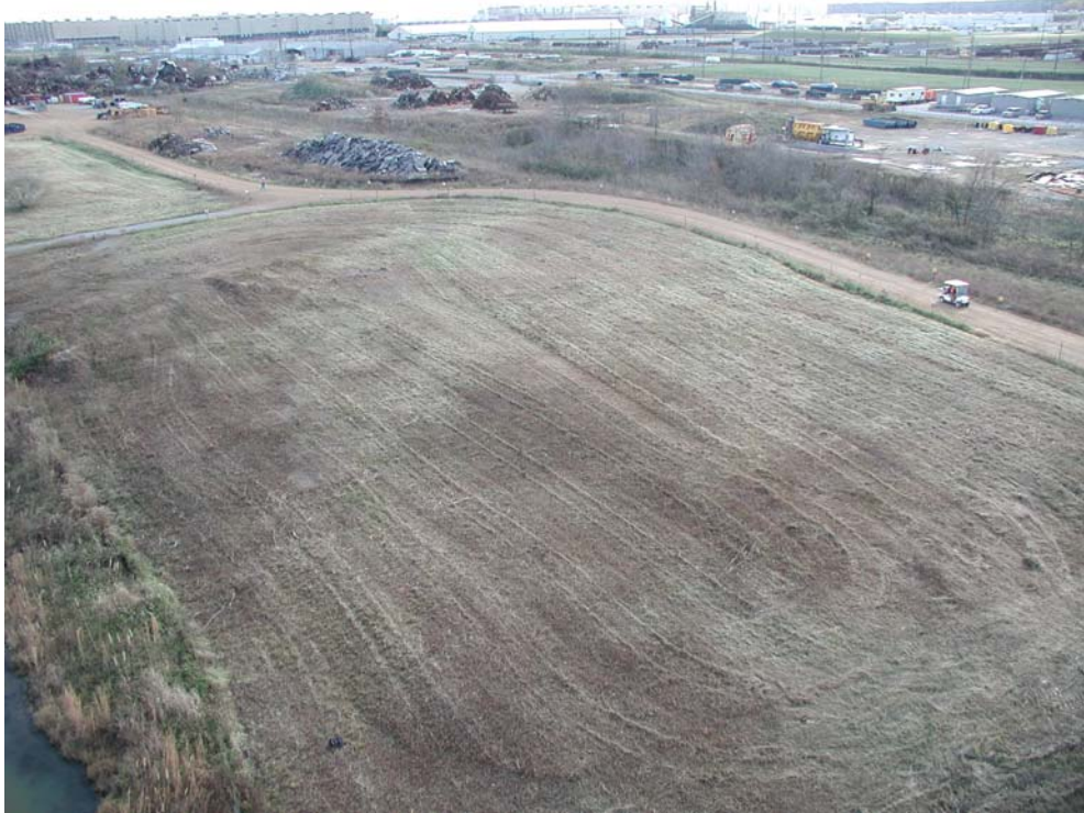
Figure G.8. SWMU 30 (Foreground, SWMU 7 Is in Upper Left)
