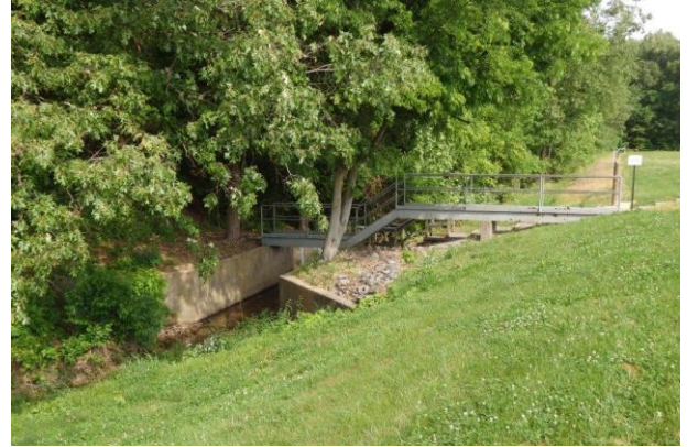
Figure 2.1. KPDES Outfall K017
