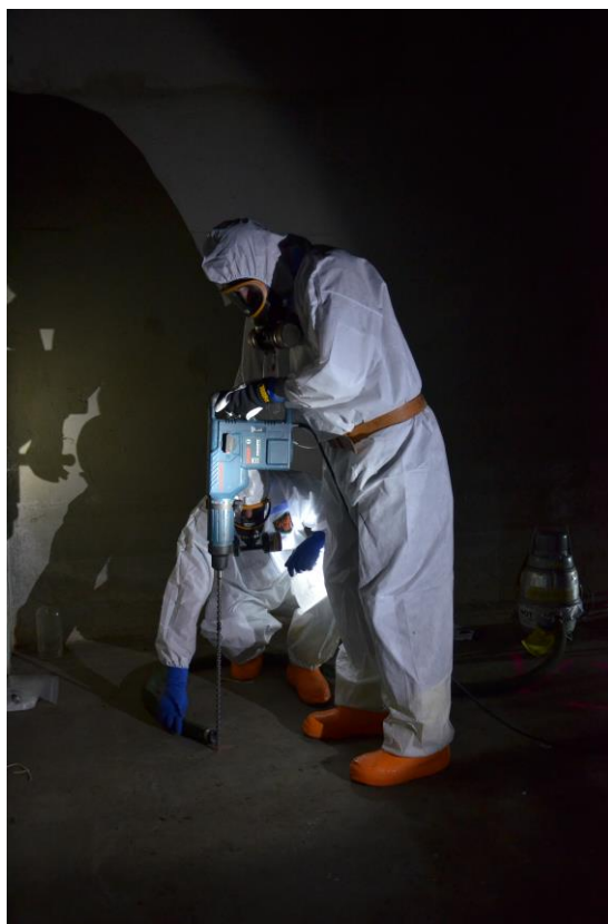
Figure 3.2. Installation of Vapor Intrusion Sampling Port
