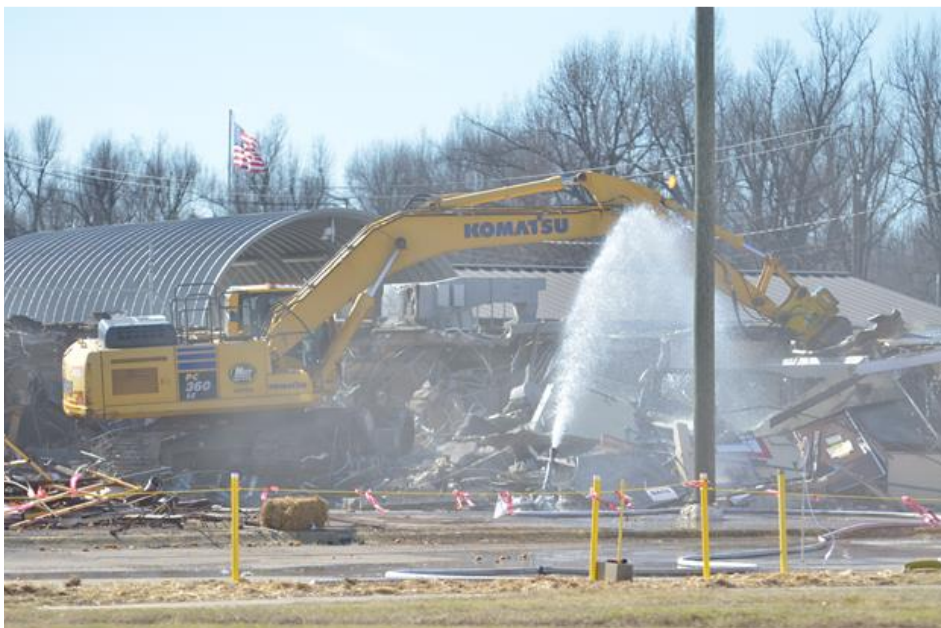
Figure 2.2. C-212 Office Building Demolition
