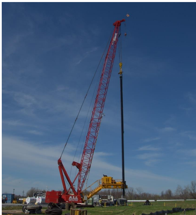
Figure 3.1. Deep Soil Mixing
