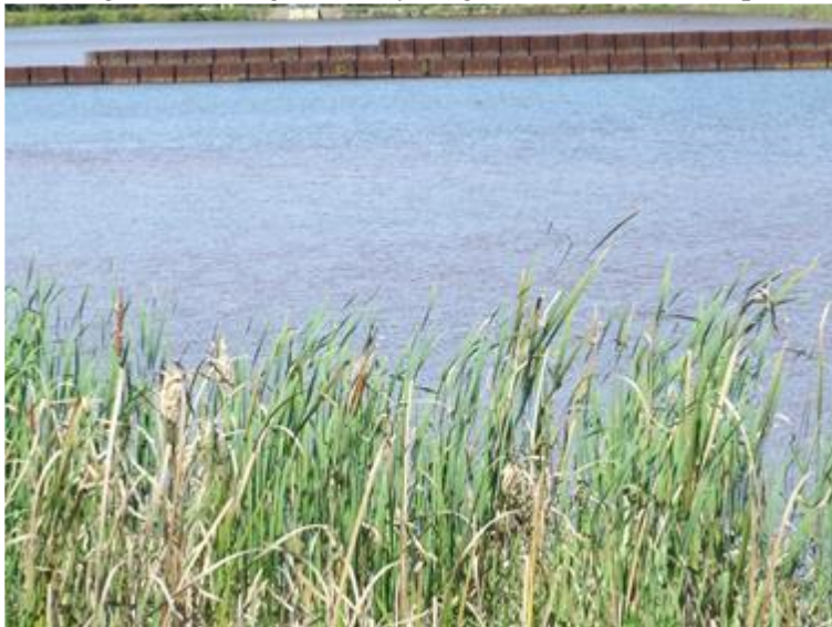
Figure 4.4. C-616 Wastewater Treatment Facility Lagoon
