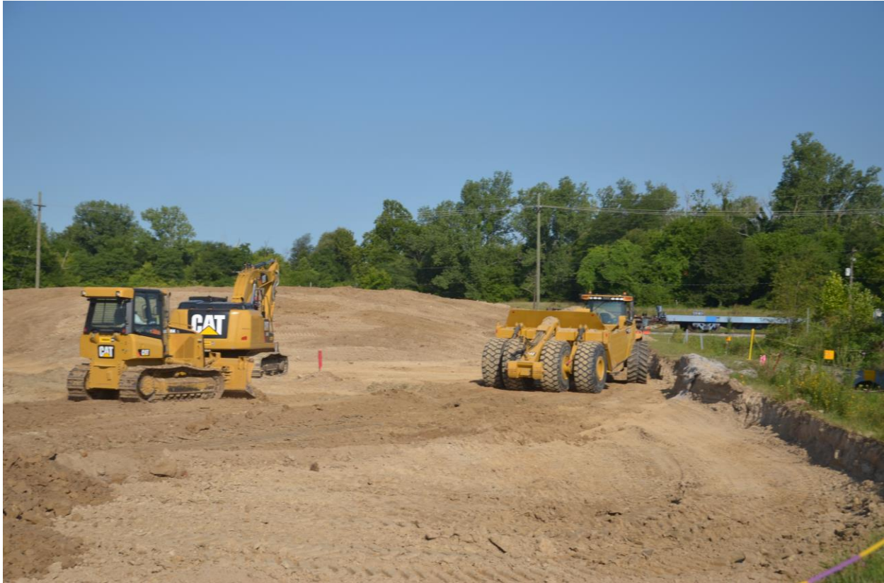
Figure 6.6. Site Preparation for Implementation of Southwest Plume SWMU 1 (Soil Mixing) Remedial Action
