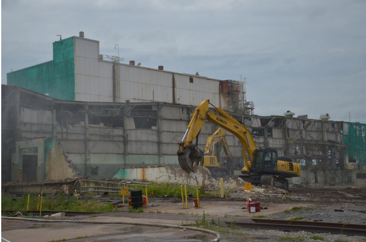
Figure 3.1. D&D of the C-410/C-420 Feed Plant Complex
