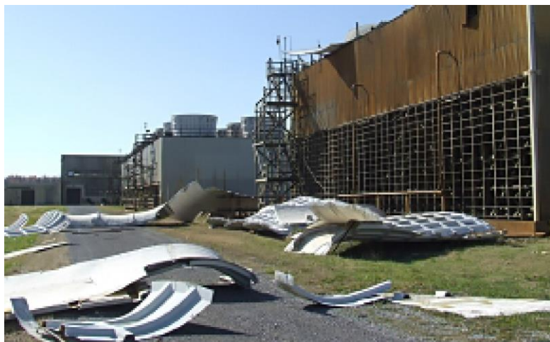
Figure 3.1. Cooling Tower Damage Sustained during 2013 Tornado
