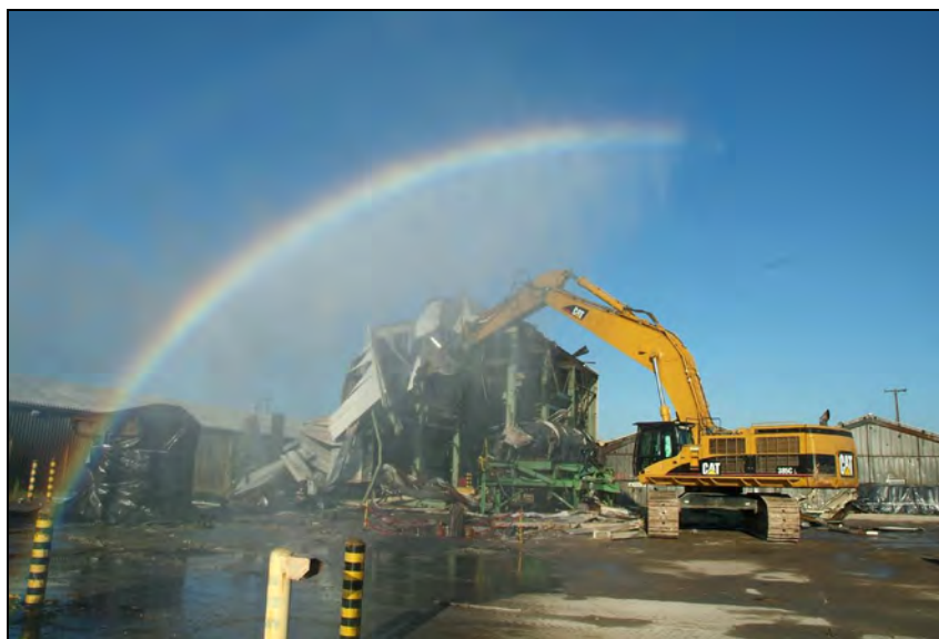
Figure 3.1. East End Smelter Demolition
