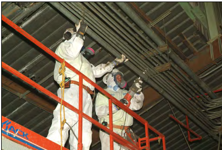
Figure 4.1. Demolition at C-746-A East End Smelter
