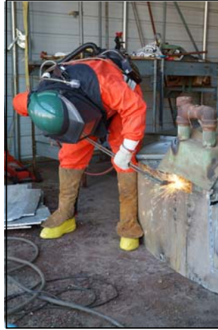
Figure 4.1. Metal Size Reduction at C-301 DMSA OS-12
