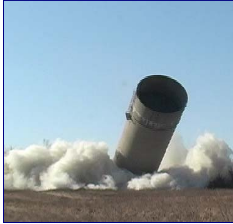
Figure 3.1. C-611 Water Tower Demolition
