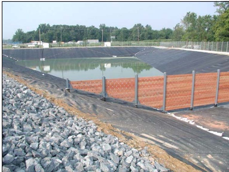
Figure 4.3. C-613 Sedimentation Basin
