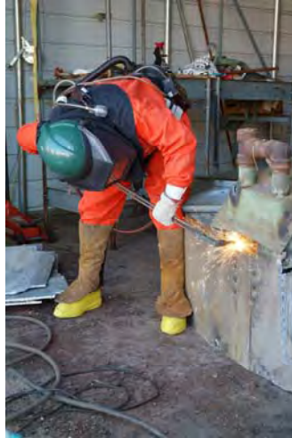
Figure 4.1. Metal Size Reduction at C-301 DMSA OS-12
