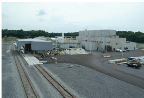
Figure 3.2. \text{DUF}_6 Facility Construction Activities
