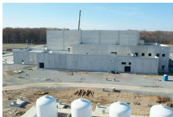
Figure 3.2. DUF 6 Facility Construction Activities
