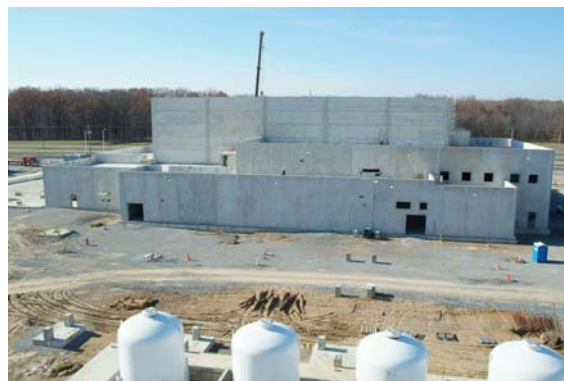
Figure 3.2. DUF 6 Facility Construction Activities
