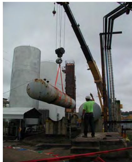
Figure 3.6. C-603 Tank Removal
