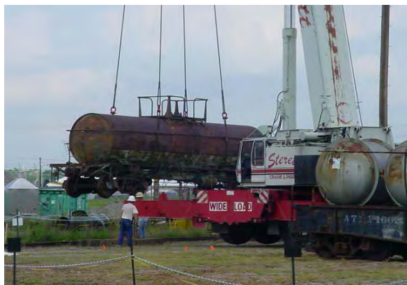
Figure 3.7. Removal of Railcar
