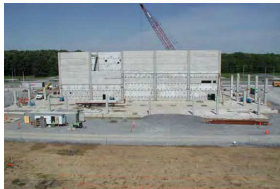
Figure 3.5. \text{DUF}_6 Facility Construction Activities
