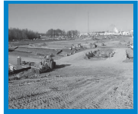
DUF 6 facility construction activities
