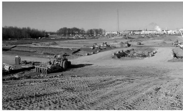
Figure 3.4 \text{DUF}_6 facility construction activities
