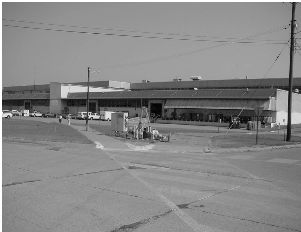
Figure 1.2 C-720 Maintenance Shop at the PGDP
