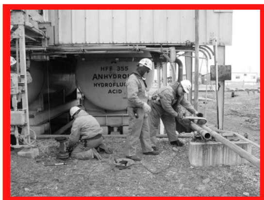
C-410 Tank Farm decontamination and decommissioning included removal of piping, structures, and tanks
