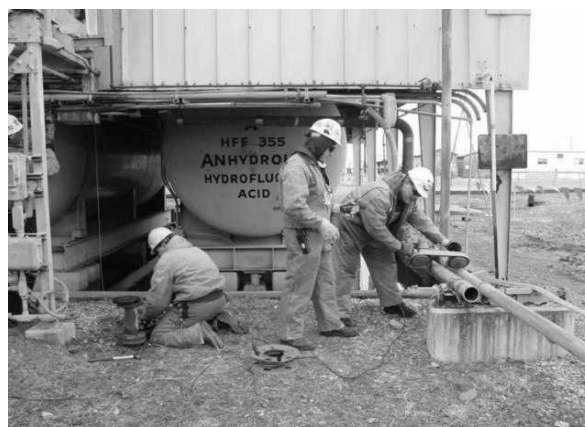
Figure 3.8 D&D of the C-410 Tank Farm included removal of piping, structures, and tanks
