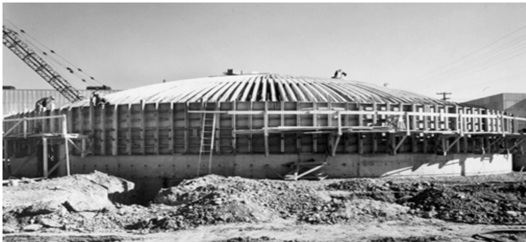
C-300 Control Center building under construction.
