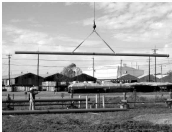
Figure 3.5 Installation of piping at the North-South Diversion Ditch.
