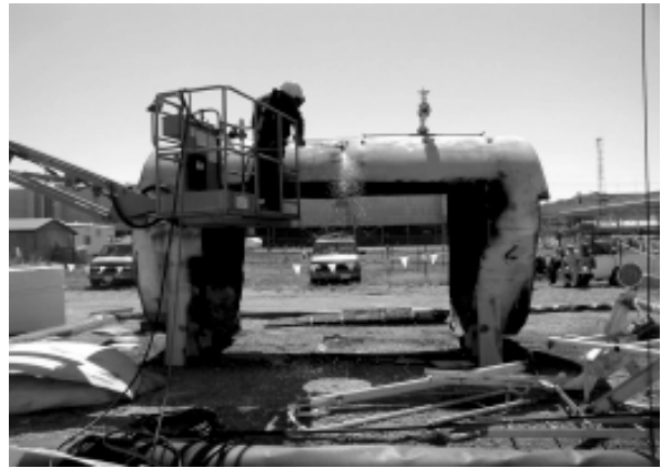
Figure 3.8 Sulfuric acid tank removal
