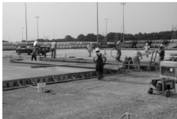
Figure 3.7 DUF 6 cylinder storage yard construction.
