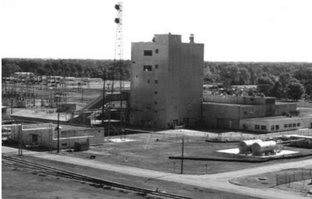
Figure 1.4 C-340 at the Paducah Gaseous Diffusion Plant.
