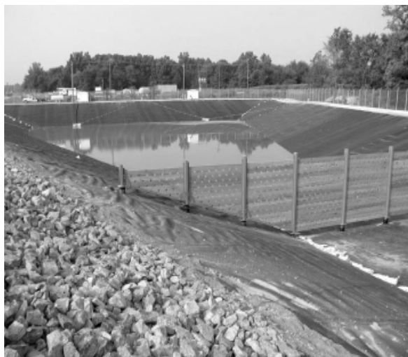
Figure 3.6 Scrap yard storm water control basin.
