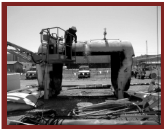
Sulfuric acid tank removal.
