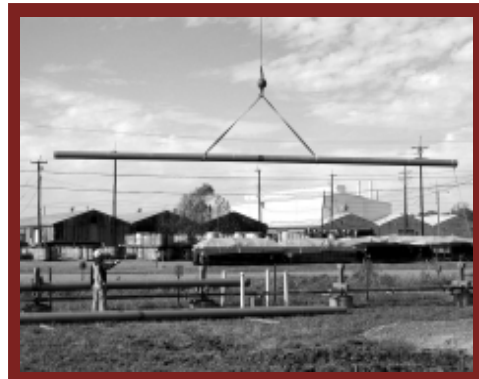
Installation of piping at the North-South Diversion Ditch.
