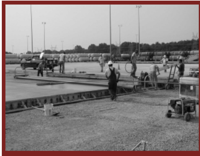
DUF 6 cylinder storage yard construction.
