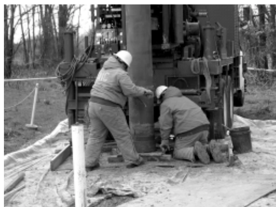
Figure 9.8 Monitoring well installation.
