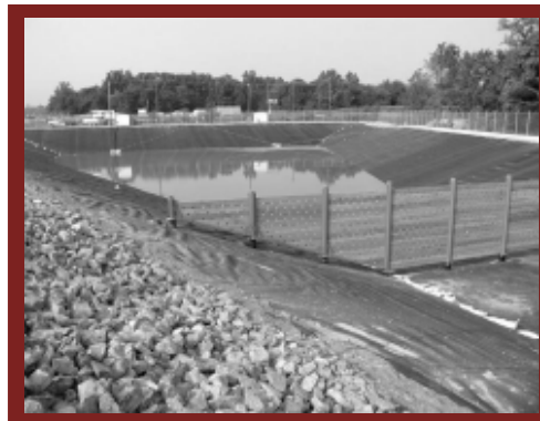
Scrap yard storm water control basin.
