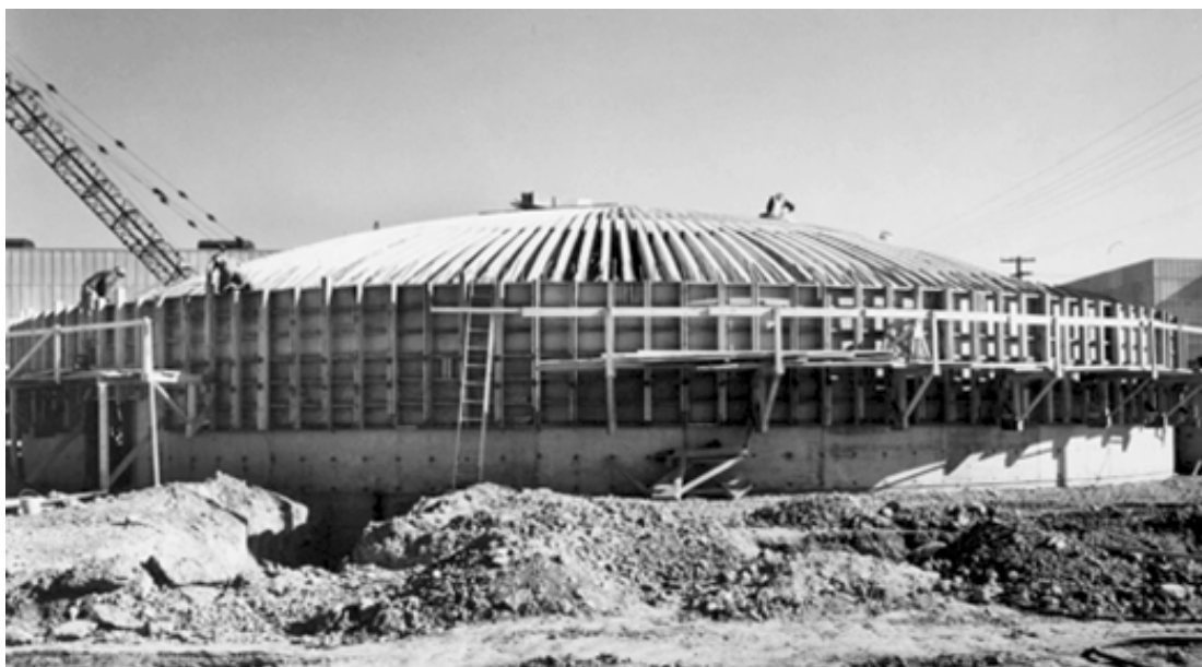
Figure 1.1 Construction of the Paducah Gaseous Diffusion Plant.
