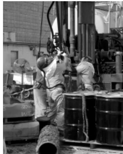
Figure 3.3 Six-Phase Heating Treatability Study system installation.
