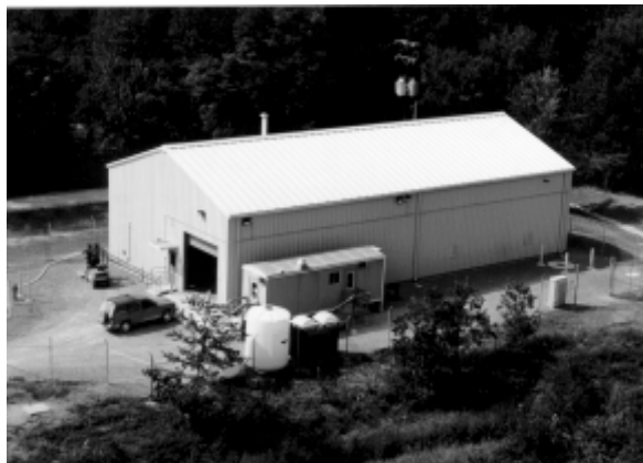
Figure 3.4 Northwest Plume Groundwater System Facility.
