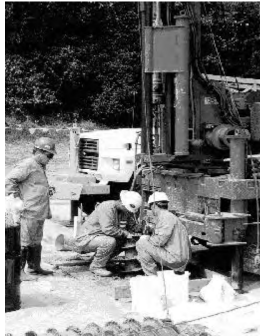
Figure 3.4 Installation of PTZ injection well.
