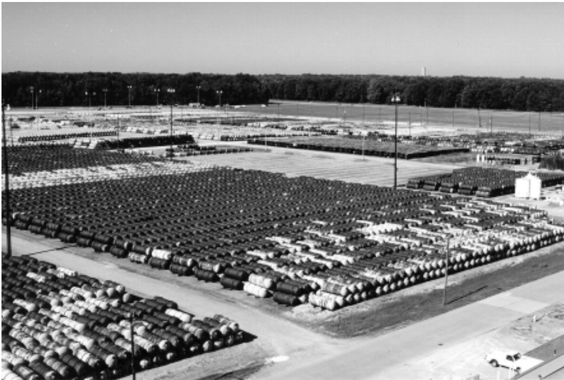
Figure 5.5 Uranium hexafluoride cylinder storage yard.
