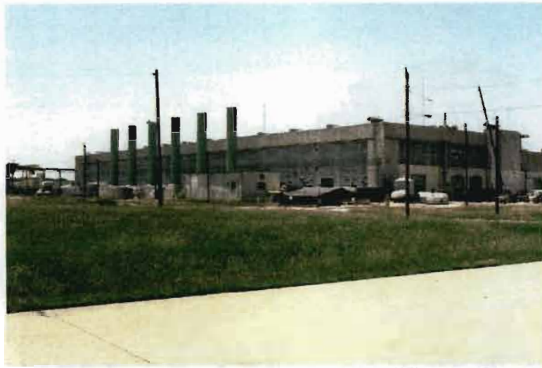
Fig. 1.4 View looking southwest toward east side of the C-400 Building—Sectors 9, 2, 3, and 4.
