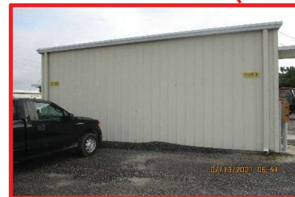
C-755-C Facility Photo: 7/2021
