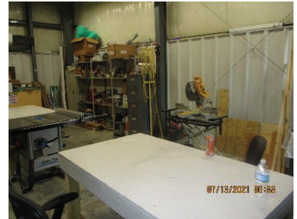
View of South Wall
