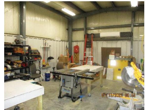
View of North and East Walls
