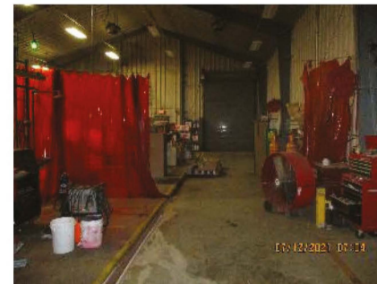
South Truck Bay Looking East
