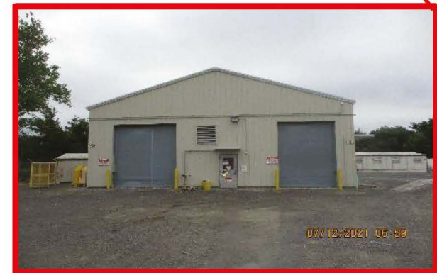
C-755-A Facility Photo: 7/2021
