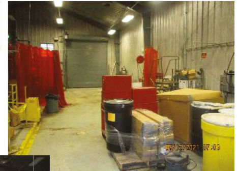
North Truck Bay Looking West
