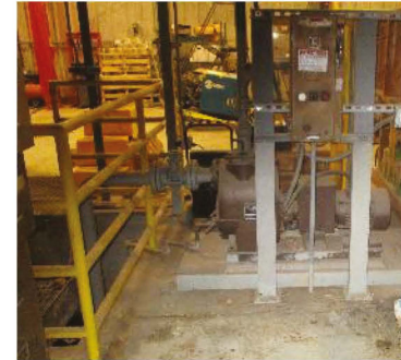
Sump Pit and Sump Pump Controls in Center Aisle
