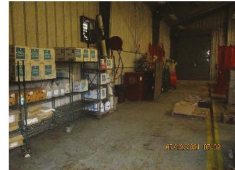
South Truck Bay Looking West
