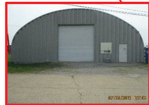
C-754-B Facility Photo: 7/2021
