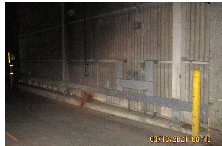
Interior south wall of C-720-J
