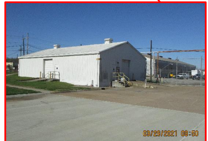
C-720-H Facility Photo: 3/2021
