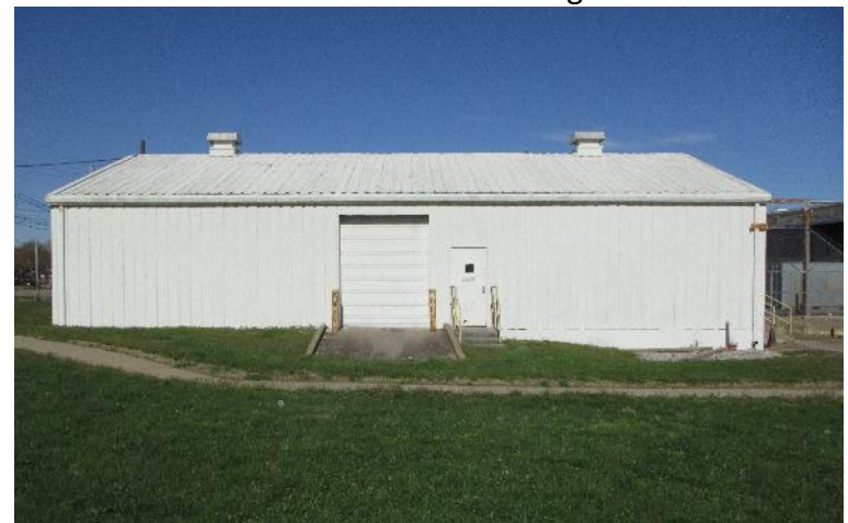
East Side of Building
