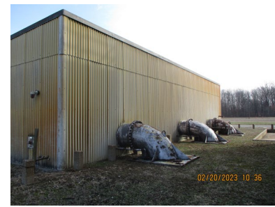
C-637-3 – Blending Pump House South Side
