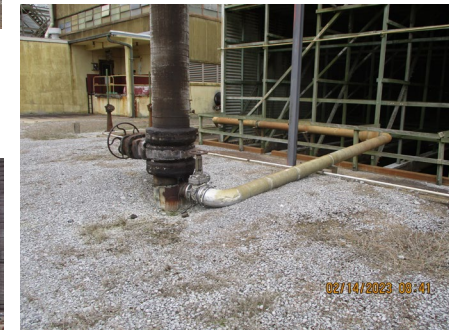
C-637-2A Cooling Tower Northeast Plume Pump and Treat Line to Riser No. 6
