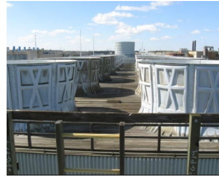
Historical Photo of Cooling Tower Roof Deck and Shrouds
