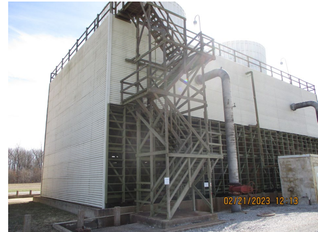
C-637-4 Northwest Corner – Stairs and Riser No. 9
