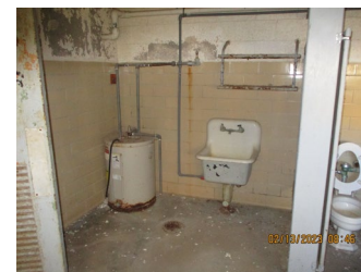
C-637-1 - East Wing Restroom/shower/change area
