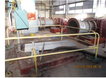
C-637-1 - Center Structure No. 3 RCW Base/Open to Wet Well
