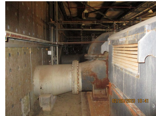
C-637-3 - Pump Suction Line Interior View
