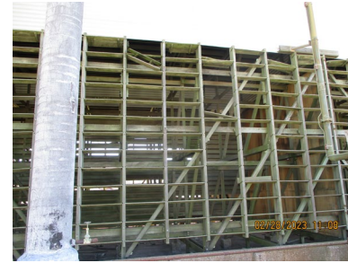
C-637-5 – Structural Frame (West Side)
