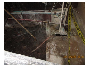
C-637-1 - West Wing Containment Area Beneath Chemical Tanks
