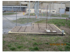
Return Crossover Vault
