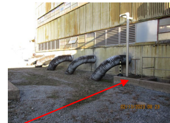
C-637-1 - Pump House Center Structure
