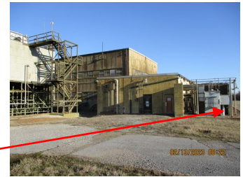
C-637-1 - Pump House East Wing View
