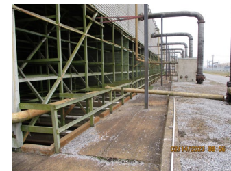
C-637-2A – West Side Concrete Roof Basin and Risers
