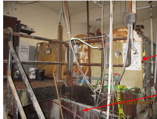
C-637-1 West Wing Diked Area beneath Corrosion Inhibitor Tanks
