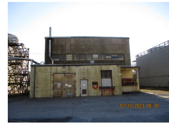
C-637-1 - Pump House West Wing View
