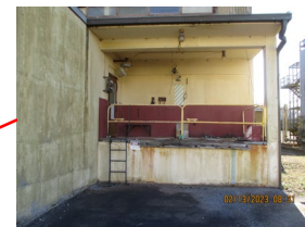
C-637-1 – West Wing Sulfuric Acid Dock
