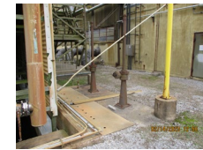
Flume/Sluice Gate Vault
