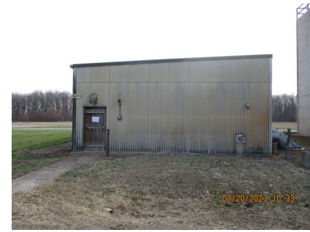
C-637-3 – Blending Pump House West Side
