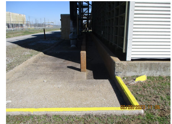
C-637-5 – West Side Roof Basin
