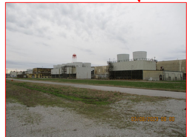
C-637 Cooling Tower Photo: 3/2023
