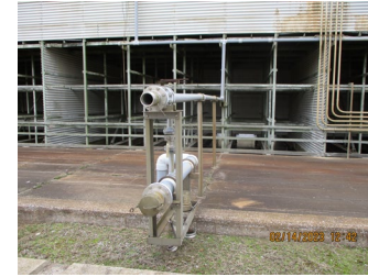
C-637-2B - Lateral Flush Line Connection Point
