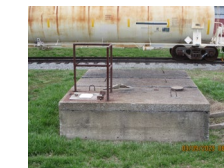
Former HPFW Vault
