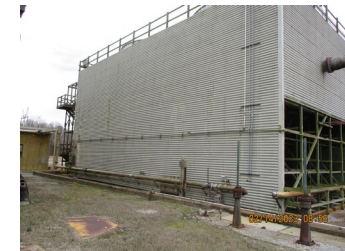
C-637-2A – North End (Sluice Gates)
