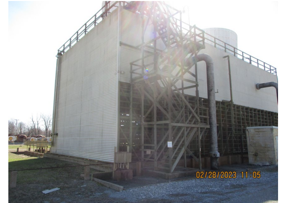
C-637-5 – West Side Stairs and No. 8 Riser
