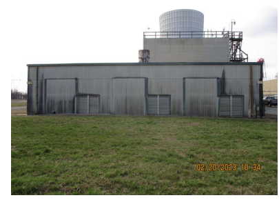
C-637-3 – Blending Pump House North Side
