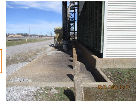
C-637-4 – West Side Roof Basin
