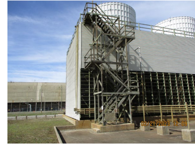
C-637-4 Southeast Corner Stairs
