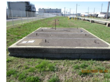
Plant Water Valves Vault
