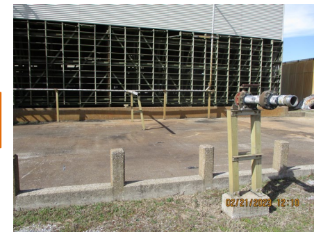
C-637-4 – Flush Line (Air-gapped)
