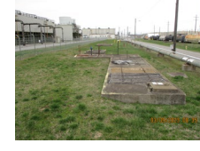
H-Loop Return Bypass/H-Loop Return/H-Loop Supply Vault
