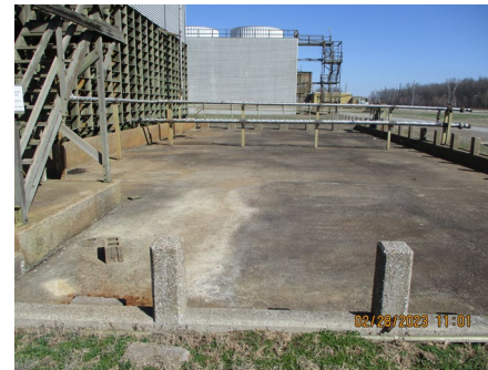
C-637-5 – Basin Roof (East Side)
