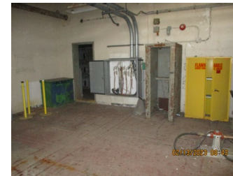
C-637-1 - Center Structure Northeast Corner
