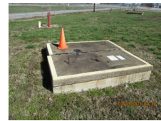
G-Loop Return Blending Tower Crossover Vault
