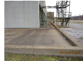
C-637-2A – South and East Side Concrete Basin Roof
