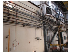
C-637-1 - Center Structure Utility Lines along West Wall
