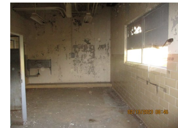
C-637-1 – East Wing Change House Locker Area
