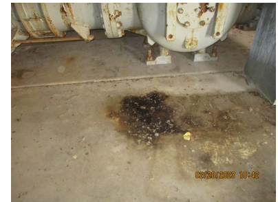
C-637-3 - Floor Staining
