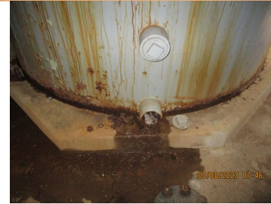
C-637-6 - Permutit® Sand Filter Tank Drain
