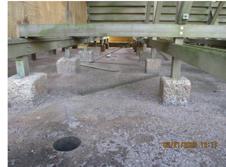
C-637-4 – Structural Frame
