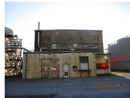
C-637-1 - West Wing Sulfuric Acid Storage and Feed Area
