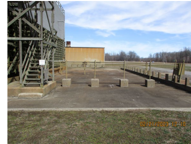
C-637-4 – East Side- Basin Roof
