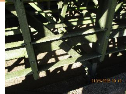
C-635-5 – Structural Frame
