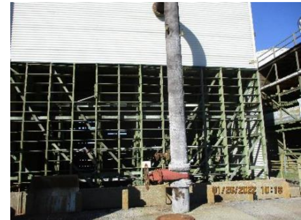
C-635-5 – East Side Riser No. 11
