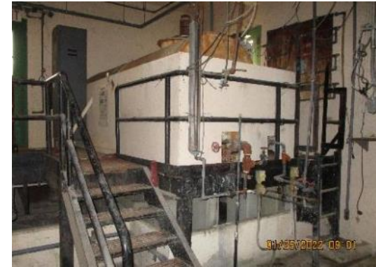
C-635-1 - West Wing Diked Area Beneath Corrosion Inhibitor Tanks
