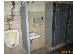
C-635-1 - East Wing Restroom/shower/change area
