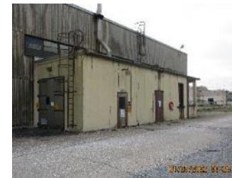
C-635-1 - Pump House West Wing
