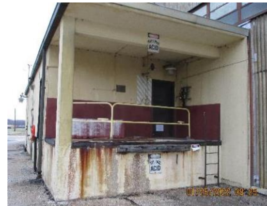
C-635-1 - West Wing Sulfuric Acid Pig and Tank Area
