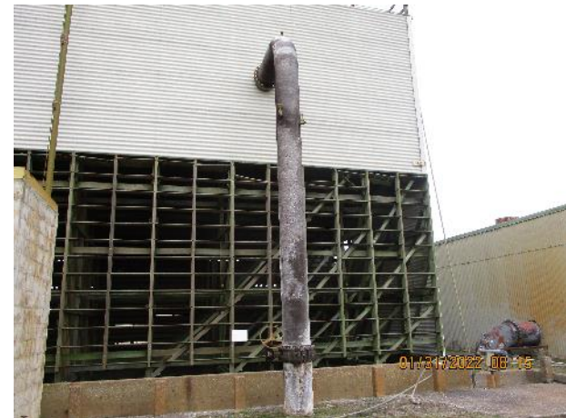
C-635-4 East Side – Riser No. 10
