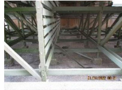
C-635-4 – Structural Frame
