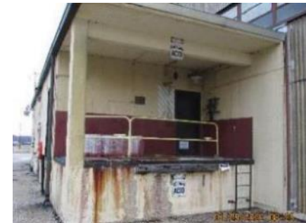
C-635-1 - West Wing Sulfuric Acid Dock
