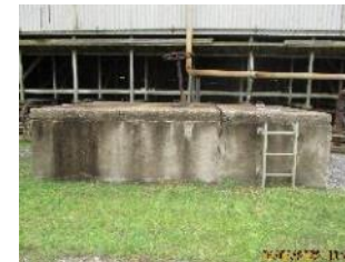
Return Cross Over Vault
