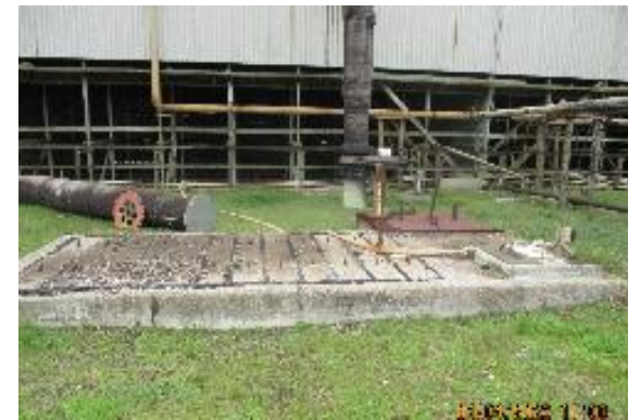
E-Loop Return and Make-up Water Vault (Valve Vault A)
