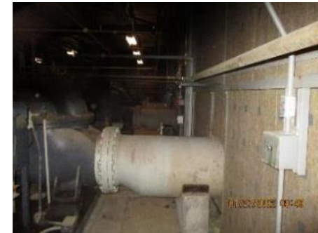
C-635-3 - Pump Suction Line Interior View
