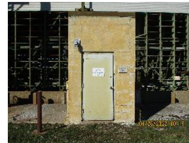
C-635-5 - Fire Sprinkler System
