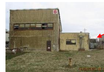
C-635-1 - Pump House East Wing
