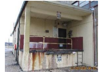
C-635-1 - West Wing Acid Platform/Loading Dock
