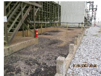
C-635-4 Basin Top – Looking South
