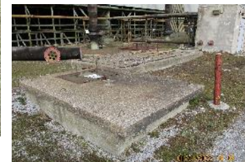
C-635-2 - Surrounding Area Vaults and Sprinkler House
