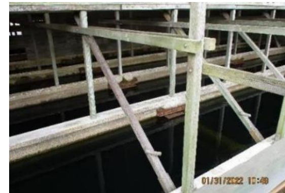
C-635-2 Cooling Tower Basin – Interior View
