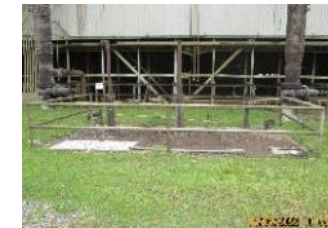
Flume/Sluice Gate/Dewatering/Tower Bypass Basin Vault
