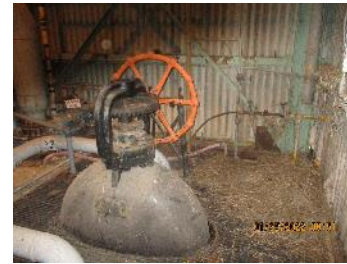
C-635-1 - Center Structure Sump (back corner)
