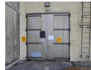
C-635-1 - West Wing North Entry Door
