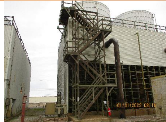
C-635-4 Southeast Corner Stairs and No. 9 Riser
