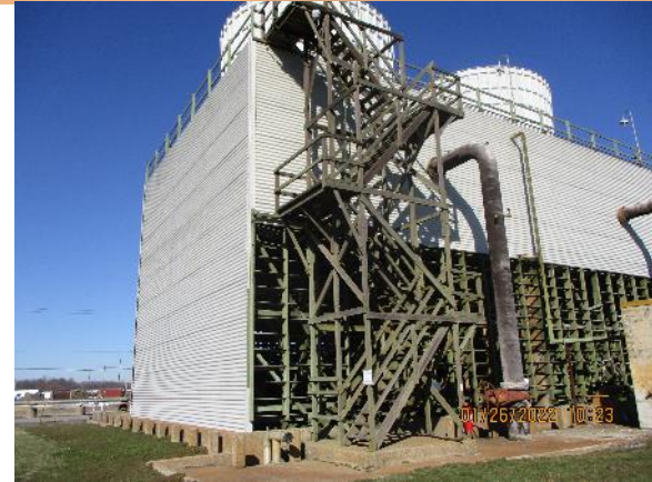
C-635-5 – Southeast Corner Stairs and No. 12 Riser
