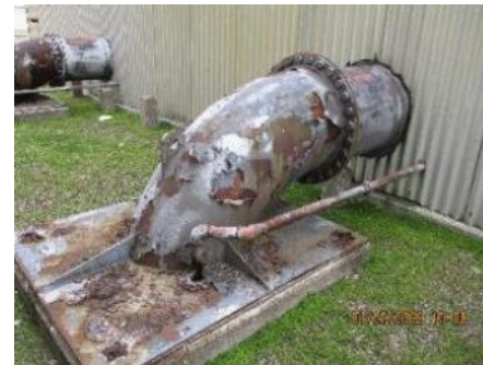
C-635-3 - Pump Suction Line Exterior View
