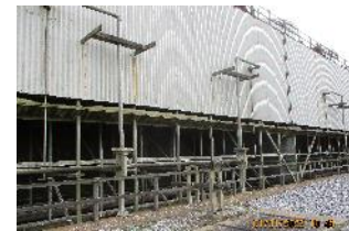
C-635-2 - Lateral Flush Lines
