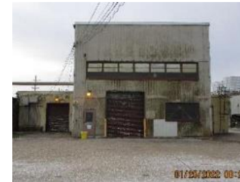
C-635-1 - Pump House Center Structure
