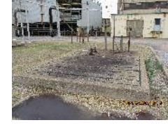
C-Loop Return Crossover Vault
