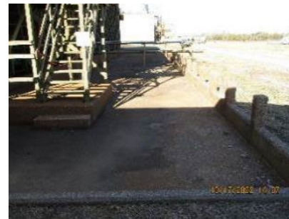
C-633-5 – East Stairway and Basin Roof
