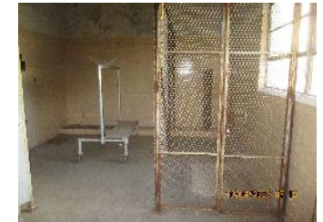
C-633-1 – East Wing Change House Locker Area
