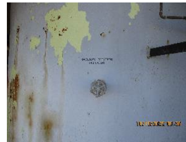
C-633-6 -Permutit® Sand Filter Tank (Backwash Rotation Indicator)
