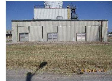
C-633-3 – Blending Pump House South Side
