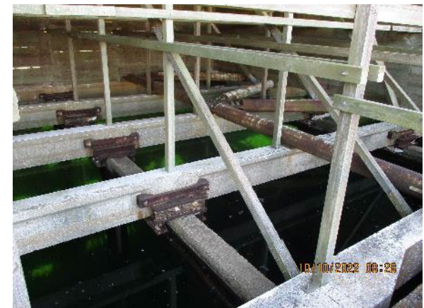
C-633-2B Cooling Tower – Interior View
