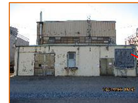
C-633-1 – West Wing Sulfuric Acid Dock
