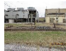
C-Loop Return/C-Loop Supply Vault
