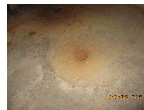
C-633-1 - West Wing Chlorine Room Floor Drain
