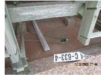
C-633-4 – Structural Frame
