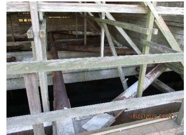
C-633-2A Cooling Tower – Interior View
