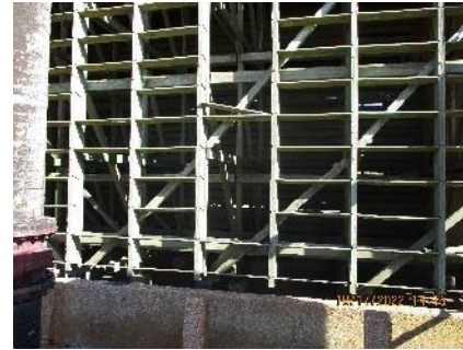
C-633-5 – Structural Frame
