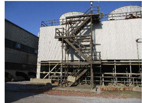
C-633-2B Cooling Tower – South East Side
