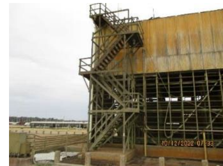
C-633-4 South East Corner Stairs
