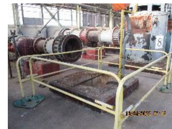
C-633-1 - Center Structure No. 9 RCW Base/Open to Wet Well
