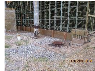
C-633-4 – Riser #9 and Manhole Cover
