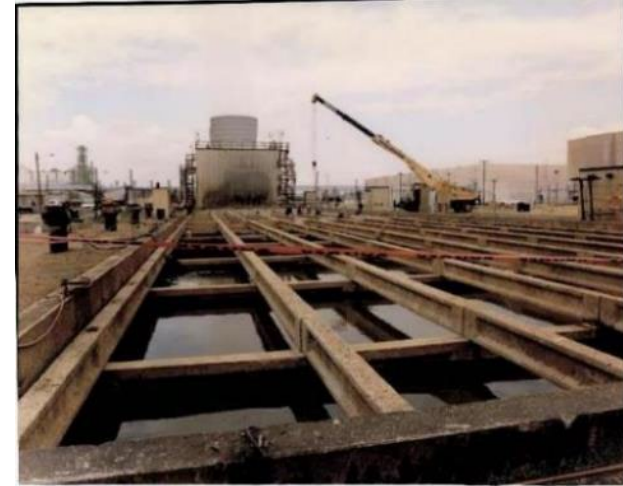
Historical photo of main cooling tower replacement project (Photo of C-633 Main Cooling Tower)
