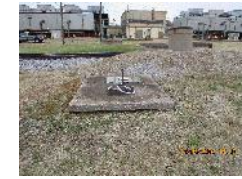
C-Loop Return to Blending Pump House Vault
