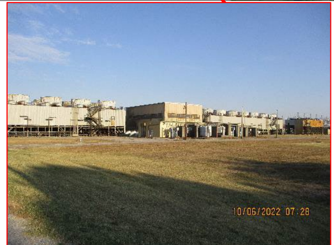
C-633 Cooling Tower Photo: 10/2022
