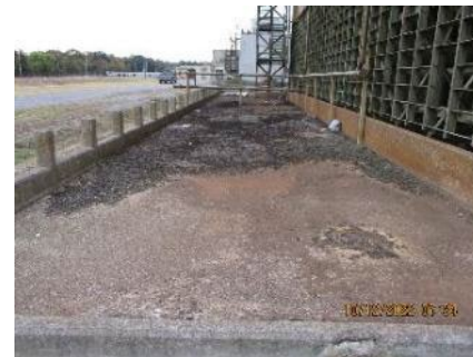
C-633-4 – East Side- Basin Roof
