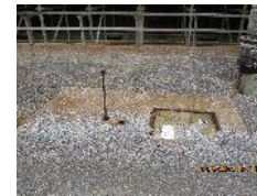
C-Loop Return Blending Tower Crossover Vault
