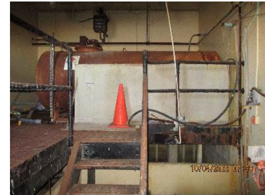
C-633-1 West Wing Diked Area Beneath Corrosion Inhibitor Tanks
