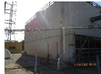
C-633-2A – North End (Sluice Gates)
