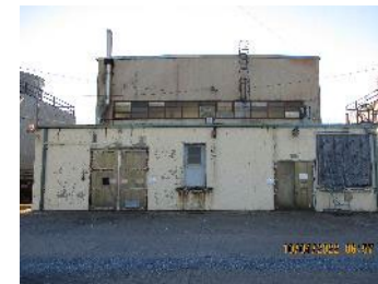
C-633-1 - Pump House West Wing View
