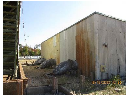
C-633-3 - Pump Suction Lines Exterior View
