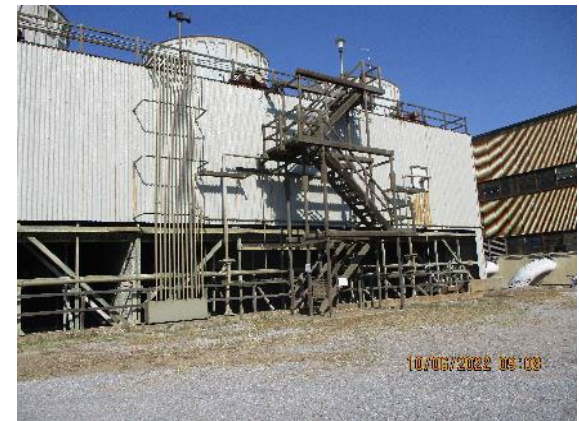
C-633-2A Cooling Tower – North East Corner
