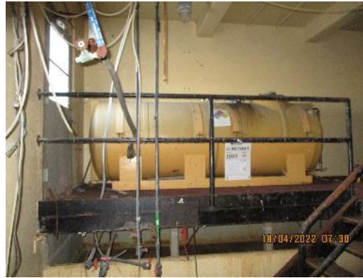
C-633-1 West Wing Diked Area Beneath Corrosion Inhibitor Tanks
