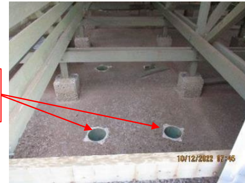
C-633-4 Top of Basin Slab
