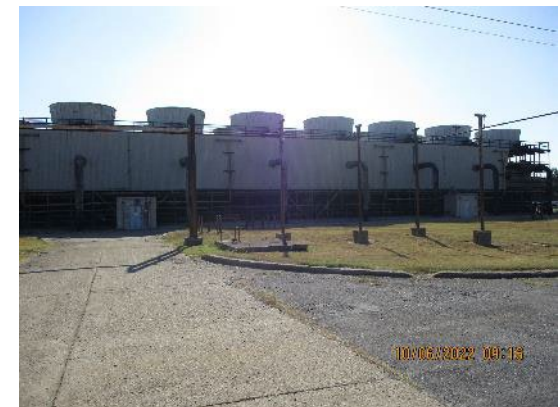
C-633-2A Cooling Tower – West Side
