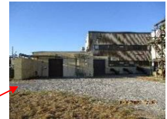
C-633-1 - Pump House East Wing View
