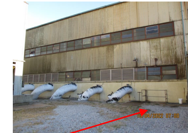
C-633-1 - Pump House Center Structure
