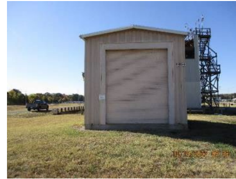
C-633-6 – Sand Filter Building North Side
