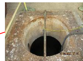
Wet Well (located beneath the concrete)
