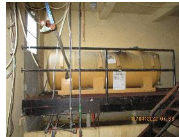
C-633-1 - West Wing Calgon Area
