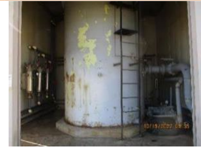
C-633-6 – Permutit® Sand Filter Tank
