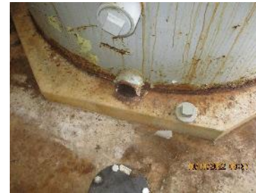
C-633-6 - Permutit® Sand Filter Tank Drain
