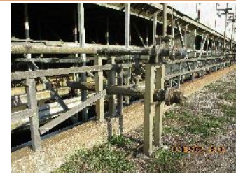
C-633-2B - Lateral Flush Line Connections
