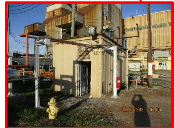
Exterior East and North Sides C-601-C Photo: 3/2021
