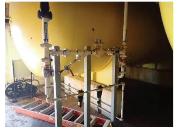
C-410-D Facility Photos: 10/2020
