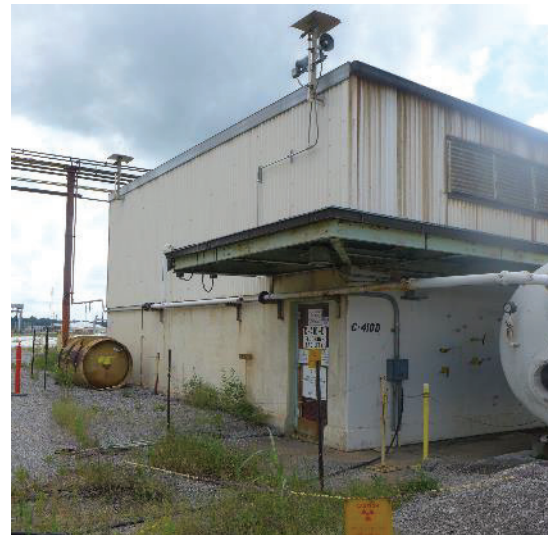
C-410-D Facility Photos: 8/2020
