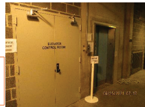
Elevator and Elevator Control Room in the Basement
