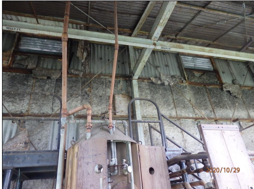
Figure 6. Interior View of the C-729 Acetylene Building
