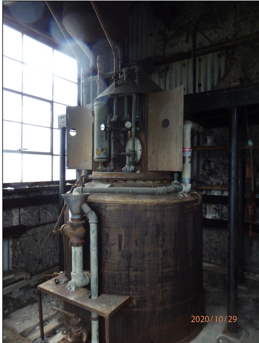
Figure 7. Interior View of C-729 Showing the Acetylene Generator
