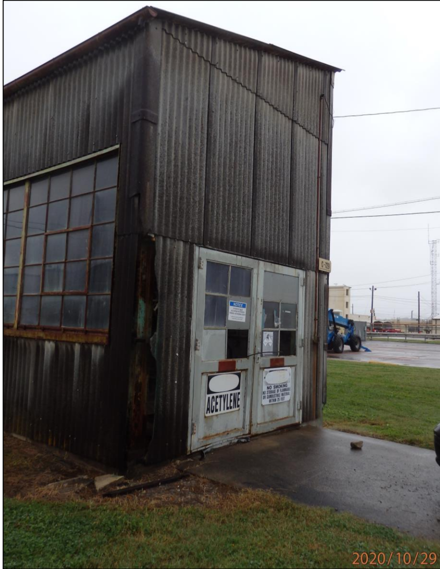
Figure 4. Exterior View of C-729 (Looking Southeast)
