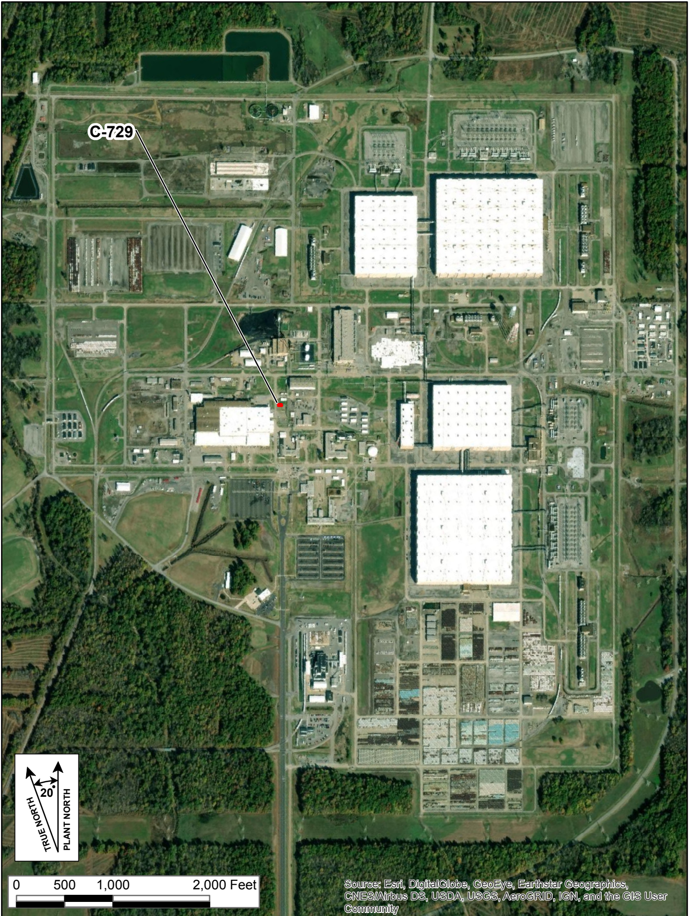
Figure 1. Aerial Photograph Showing the C-729 Acetylene Building Location
