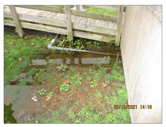
Figure 9. Standing Water in the Surface Ditch near the Sump Pump Discharge
