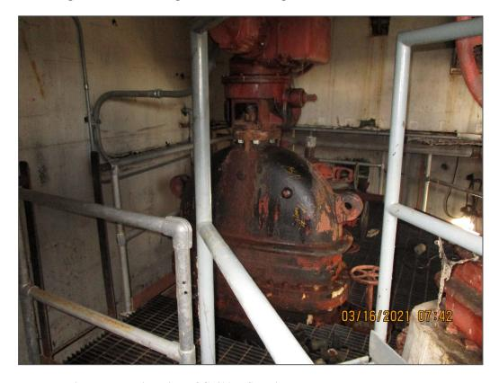
Figure 7. Interior View of C-611-T Showing the Plant Water Inlet Valve
