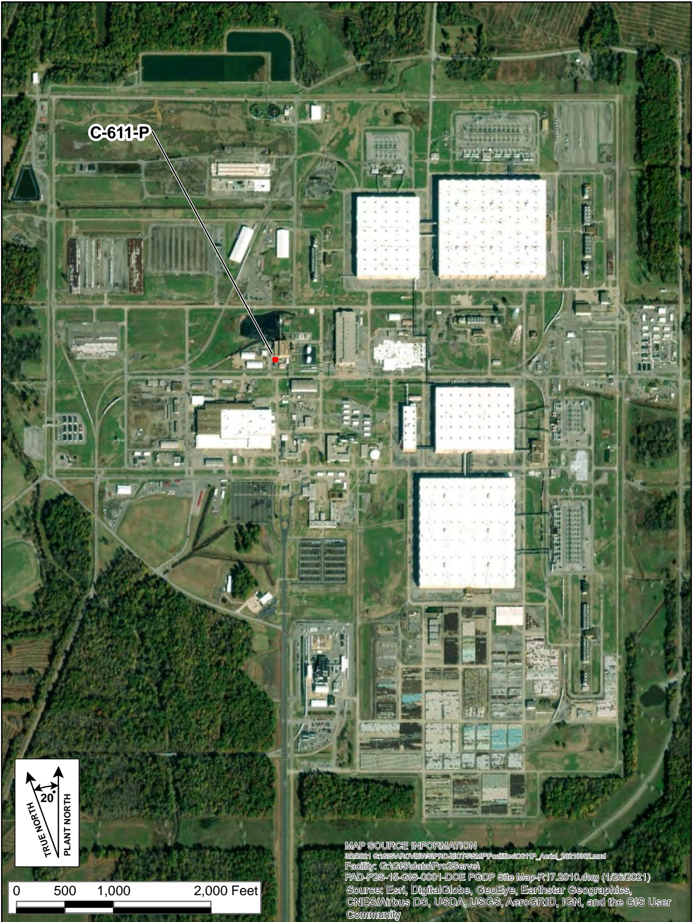
Figure 1. Aerial Photograph Showing the C-611-P Building—Pump House Location
