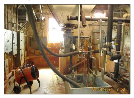
Figure 12. Ferric Sulfate Feeder System in C-611-B
