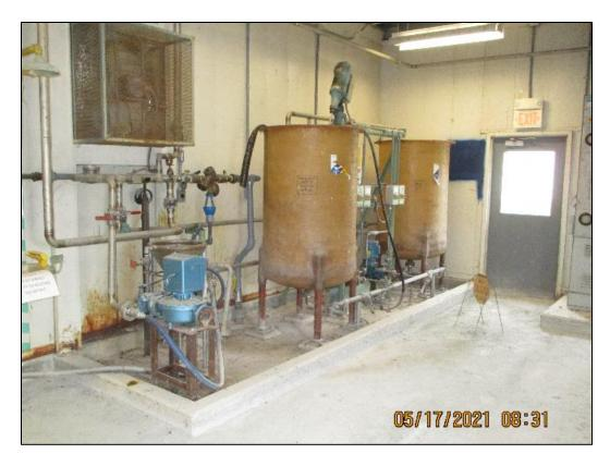
Figure 19. Interior of C-611-F2 Showing Polymer Mixing Tanks
