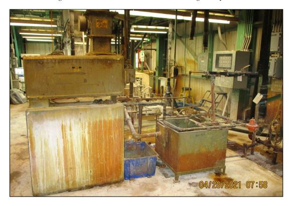
Figure 34. Ferric Sulfate Feeder and Mixing Tank in C-611-U
