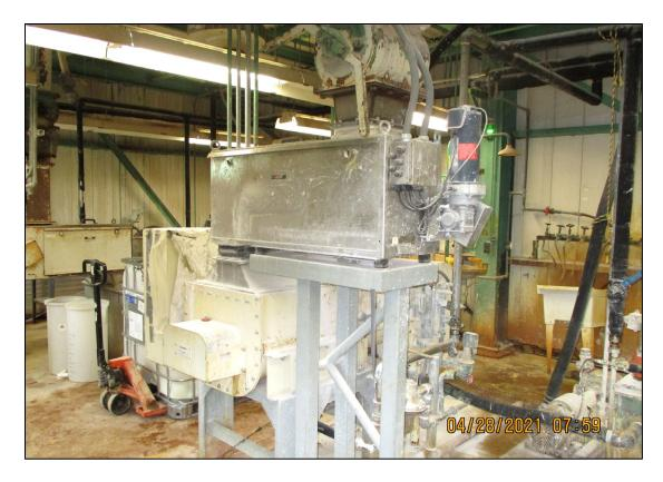
Figure 35. Lime Feeder and Slaker in C-611-U
