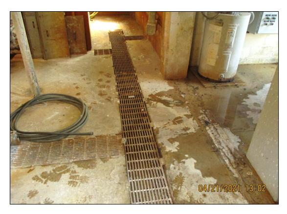
Figure 13. Floor Collection Trench in C-611-B (Leads to an Exterior Sump Pit)
