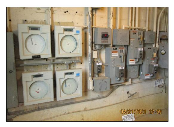
Figure 11. Water Flow Charts and Valve Controls in C-611-B
