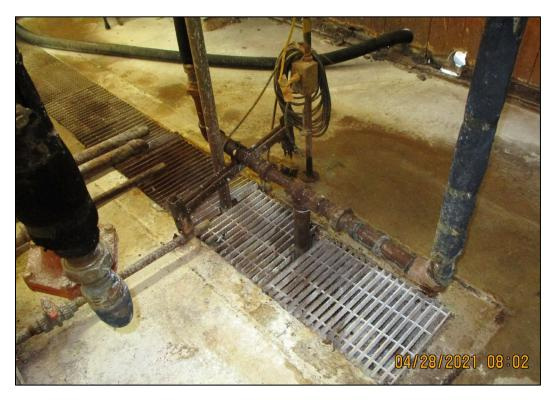
Figure 36. Floor Trench with Suction Line in C-611-U
