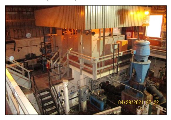
Figure 24. View of the Interior of C-611-J Showing Pumps, Piping, and Switchgear Room
