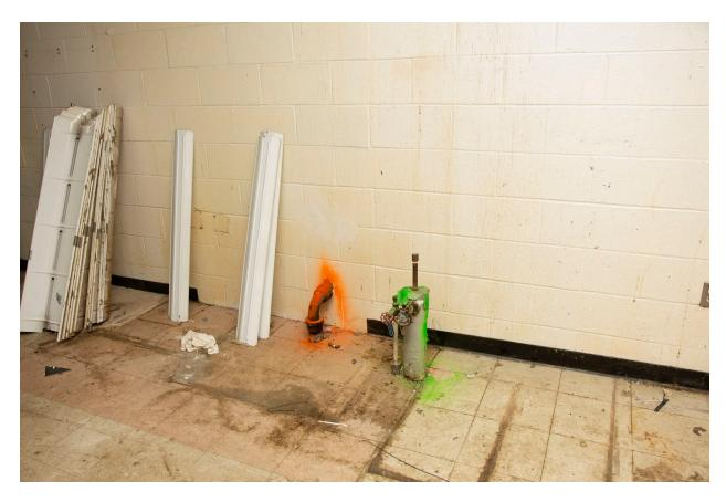
Figure 9. Roof Drain Piping Painted Orange to Identify Potential Lead Joints and Green Paint on Pipe Wrapping Indicating Non-asbestos Materials (9/2019)
