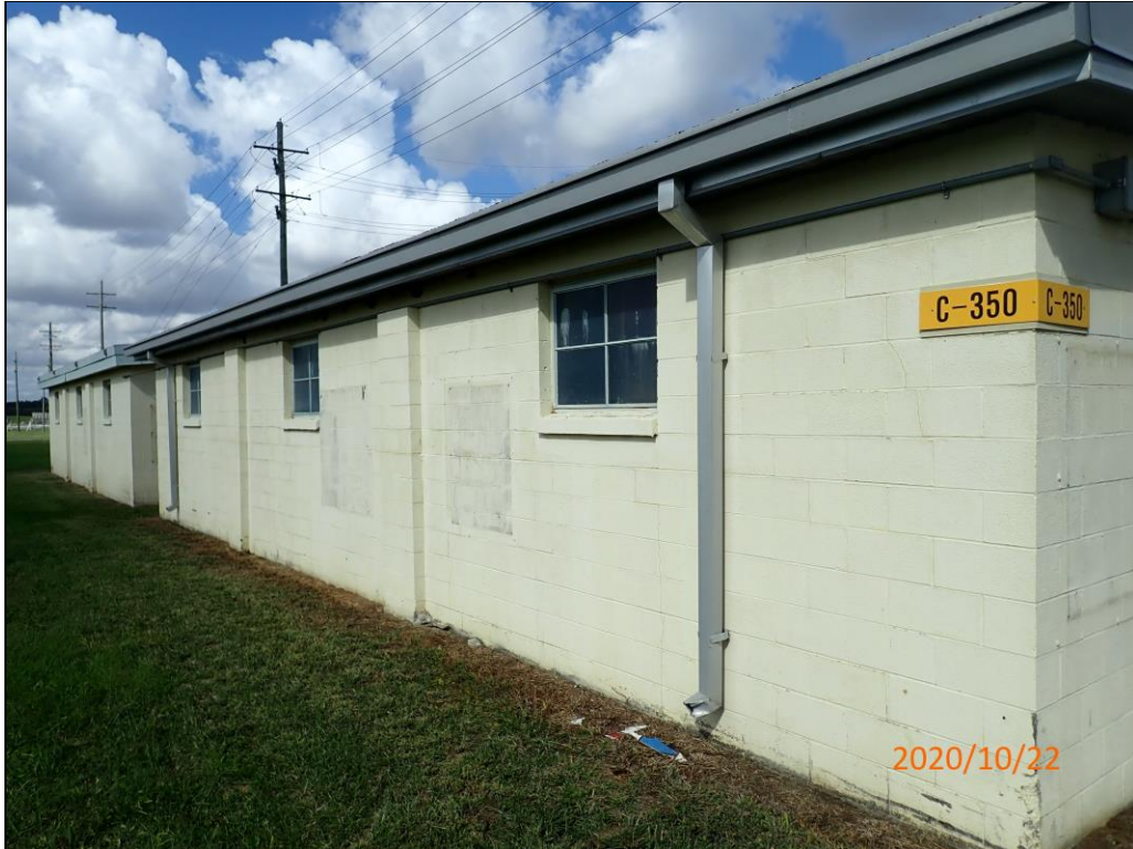
Figure 4. Exterior of C-350, Southeast Corner (Looking West)
