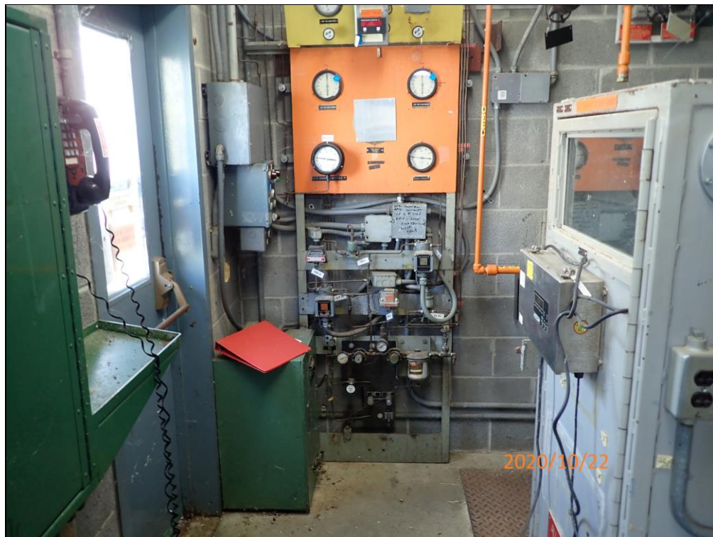
Figure 9. Inside the North Extension
