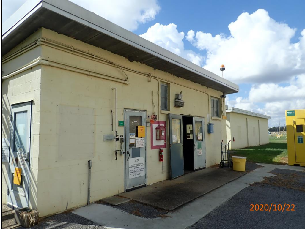
Figure 3. Exterior of C-350 (Looking South at the North Extension)
