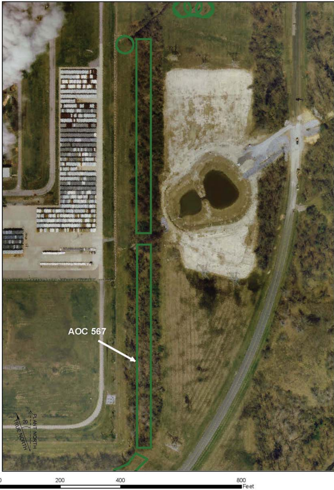
Figure E1.39. Photograph of AOC 567
