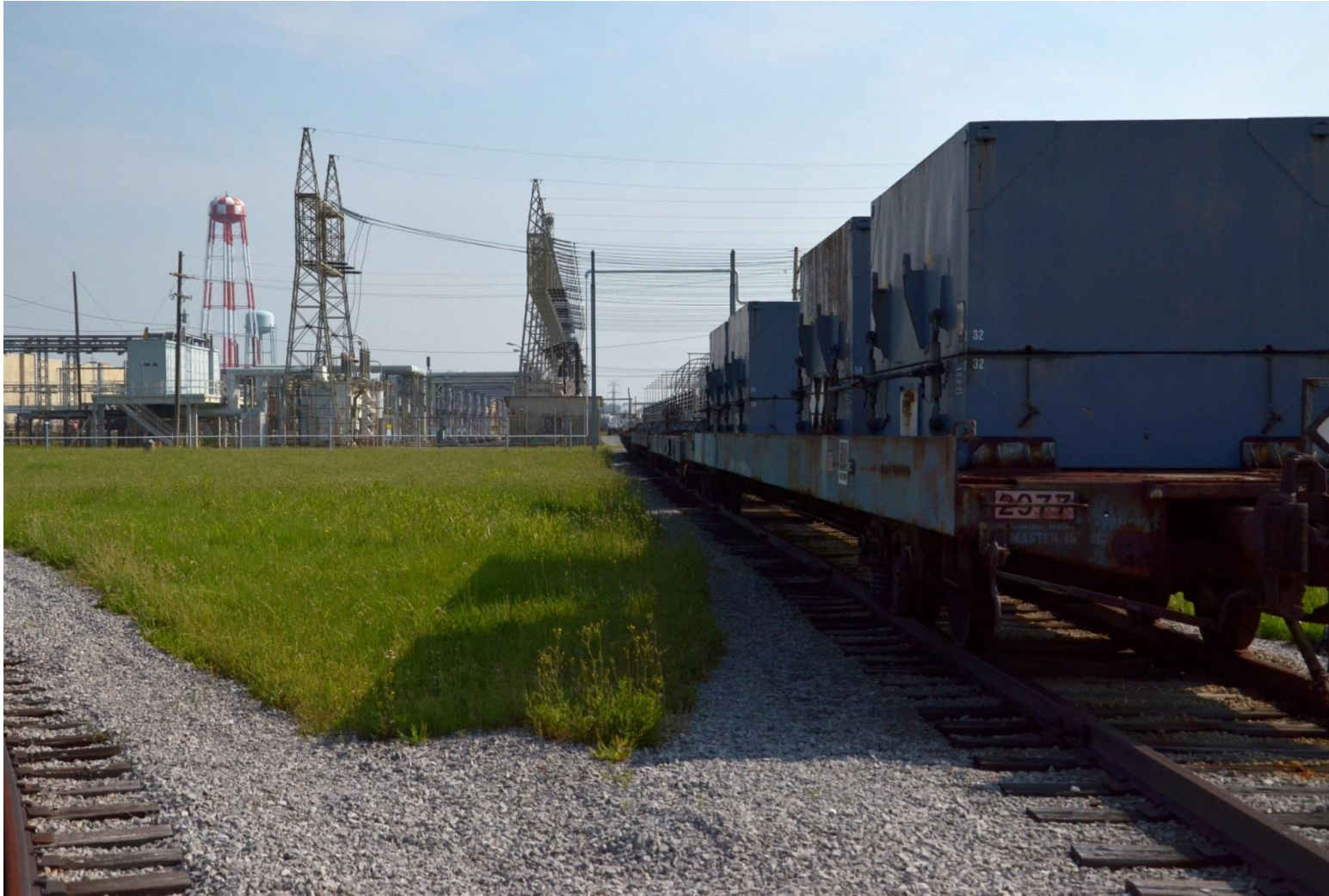
SWMU 225A (Looking North) DMSA OS-14 June 6, 2013
