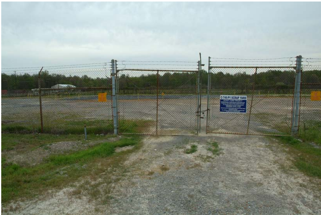
C-746-P1 Scrap Yard
