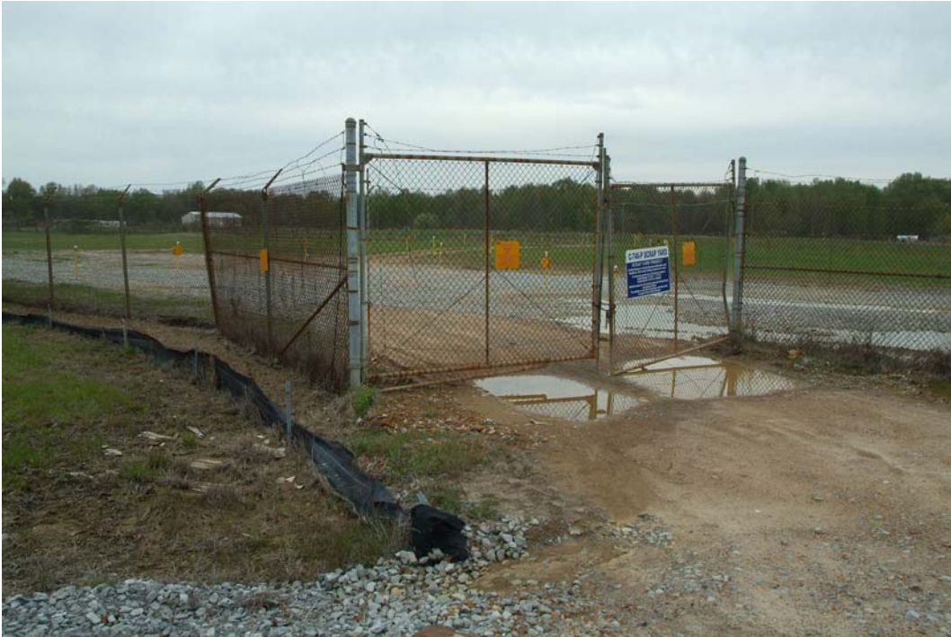
C-746-P Scrap Yard
